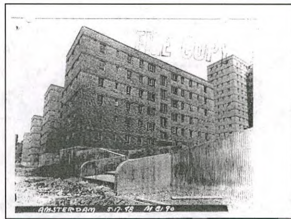
Corrugated Concrete Walled Stairway
