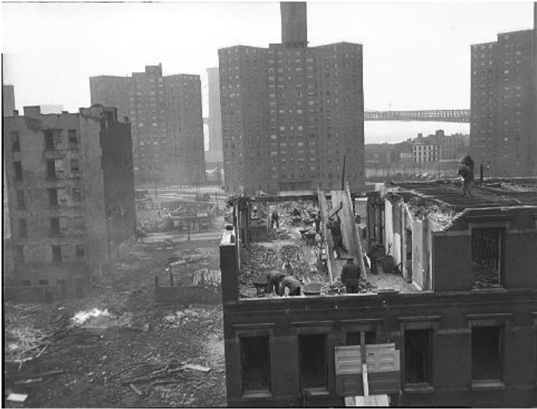
A Tenement being Demolished for Phase 2 of the Gov. Alfred E. Smith Houses, 11/27/1950. In the background Phase 1 is nearing completion, and in the far background is the Brooklyn Bridge. NYCHA started using the technique of sectional construction of slum clearance projects so that fewer families would need to be displaced at one time and new housing could be filled more rapidly (photo 02.003.13916).
