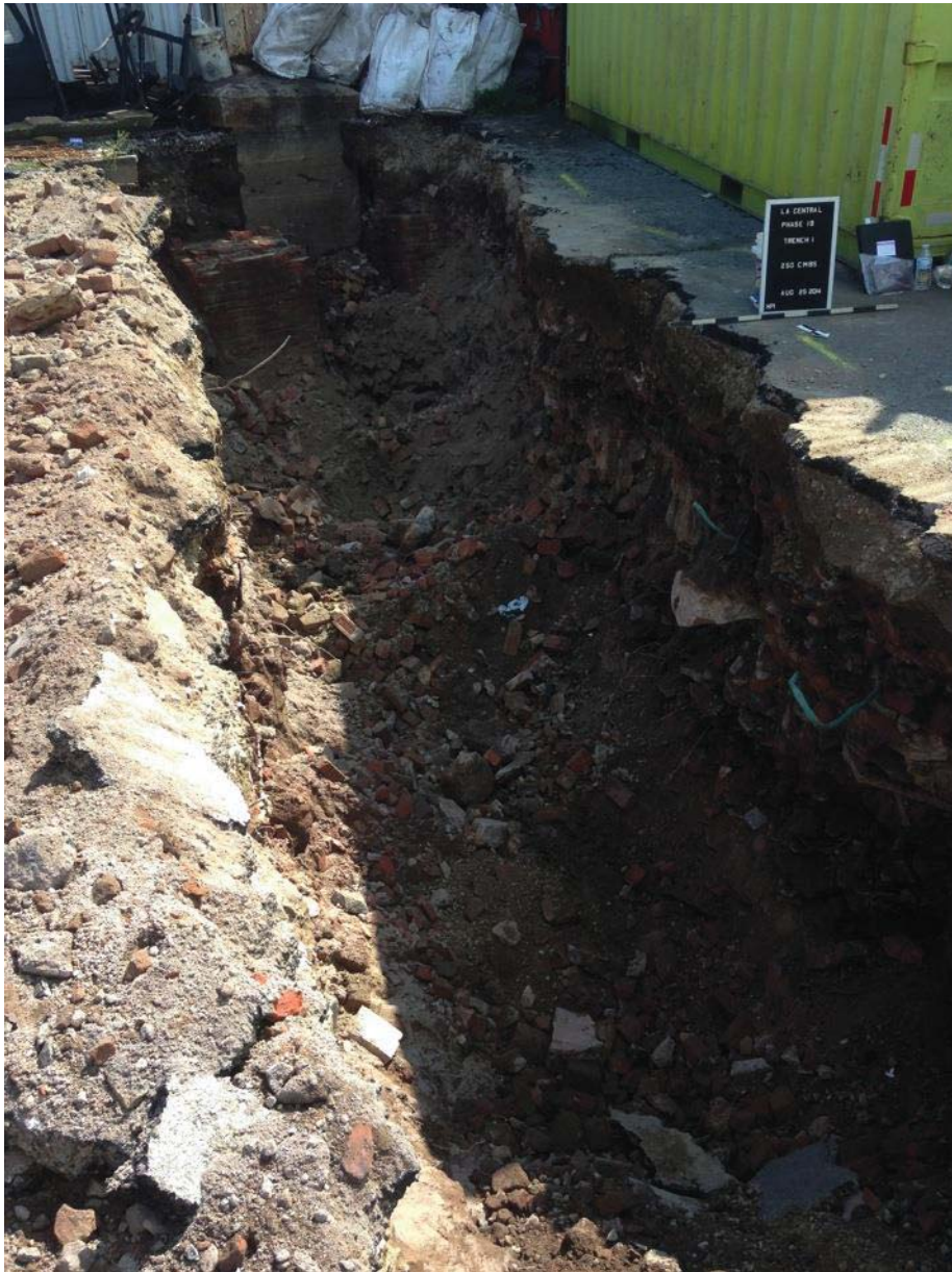
Photograph 6. Overview of Trench 1.
