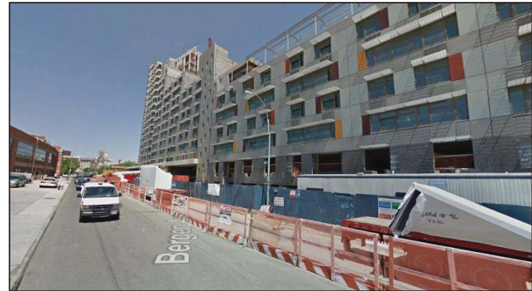
8. View looking north at Via Verde from Bergen Avenue.
