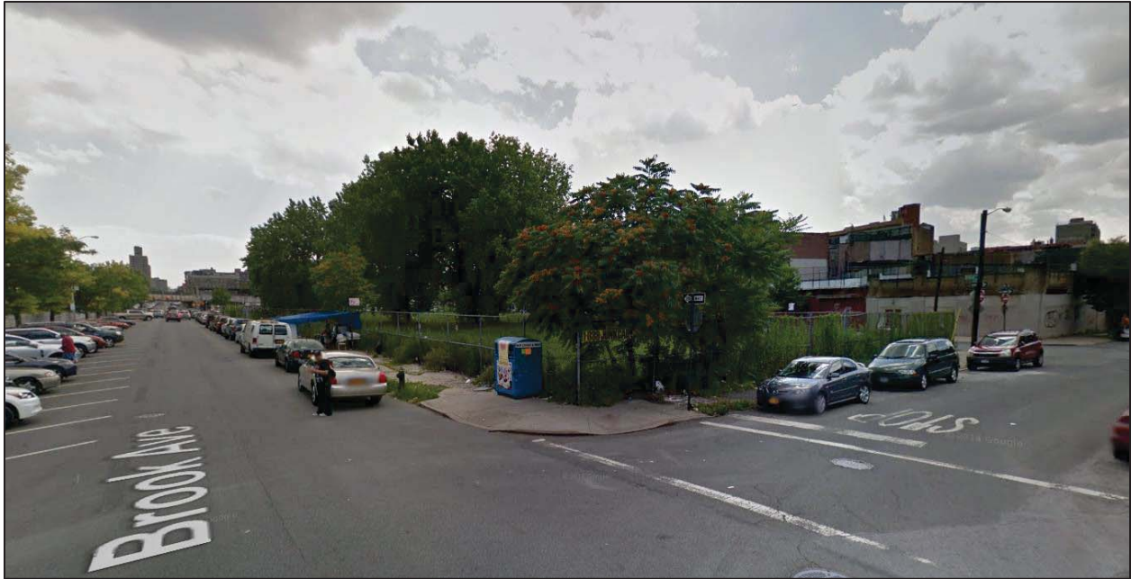
5. Existing/No-Action Conditions: View looking southwest from the intersection of Brook Avenue and East 153 rd Street, with fenced-in vacant land on the proposed development site.
