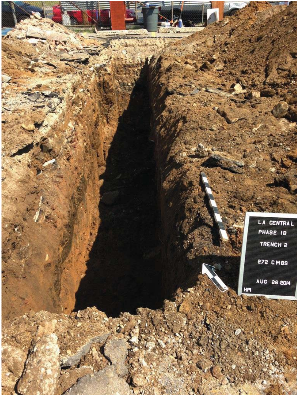
Photograph 9. Overview of Trench 2.
