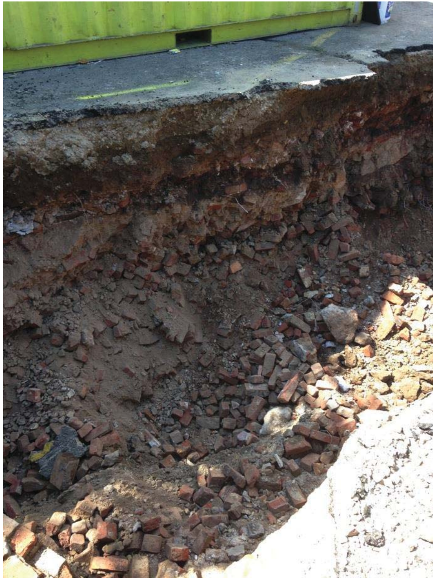
Photograph 3. Trench 1, Fill Strata.
