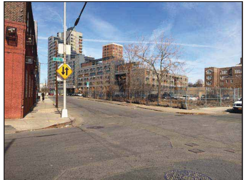
8. View looking northeast from Bergen Av./E.153rd St.
