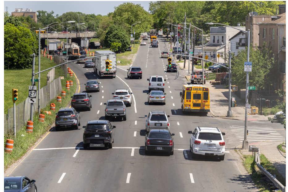
Missing sidewalks contribute to the danger of walking along or crossing Conduit Avenue
