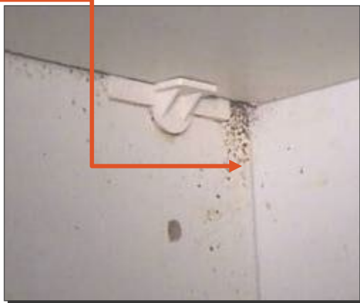
Cockroach dropping ("frass") under cabinets
