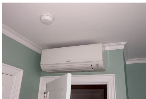
INDOOR UNITS PLACED ABOVE DOORS REDUCE RISK OF COLD AIR FALLING ON OCCUPANTS IN COOLING MODE
