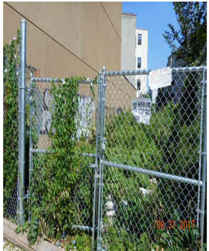
16. View of the front side of the Subject Property, along Fulton street
