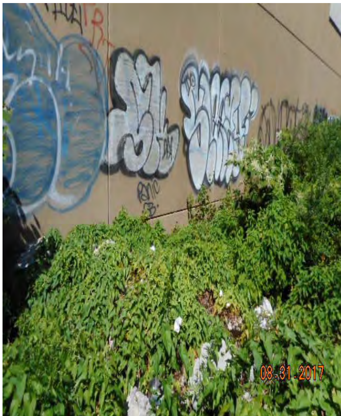
17. View of western portion of the Subject Property
