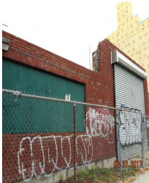
2. View of the boundary wall on the southern side of the Subject Property
