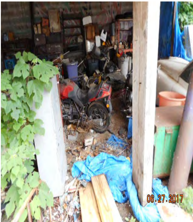
3. Storage shed-Miscellaneous debris storage
