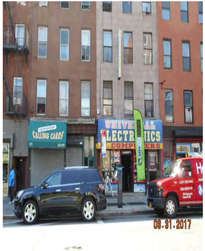
20. The adjacent properties to the south across Fulton Street
