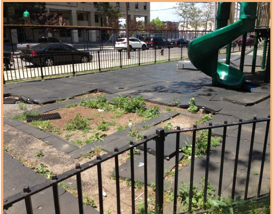
Image 5: damage concrete. Source: marktregerforcouncil.com
