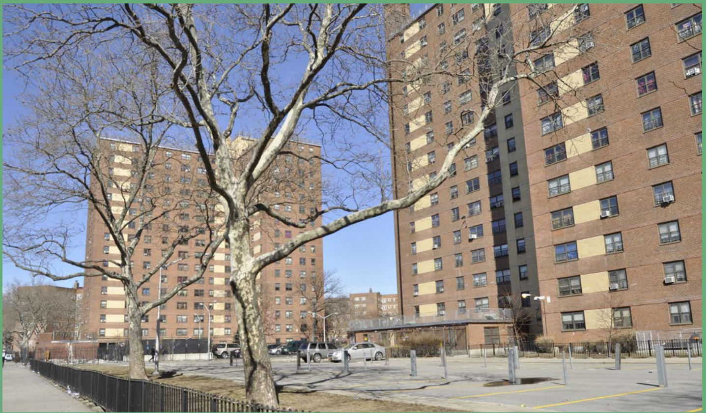
Rockaway Avenue and Livonia Avenue before infill development
