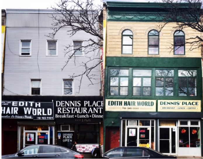
Storefront improvements of 1701 Pitkin (before and after)
