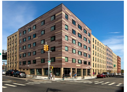
STONE HOUSE (COMPLETED)
