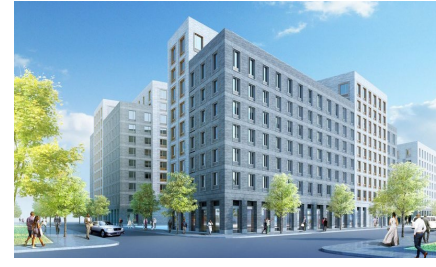
EBENEZER PLAZA (UNDER CONSTRUCTION - 2021)
