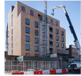
210-214 HEGEMAN AVE (COMPLETED)
