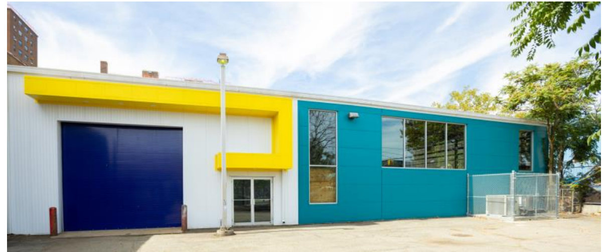
East New York Industrial Building at 181 Powell St
