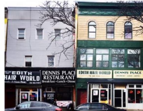
Storefront improvements of 1701 Pitkin (before and after)
