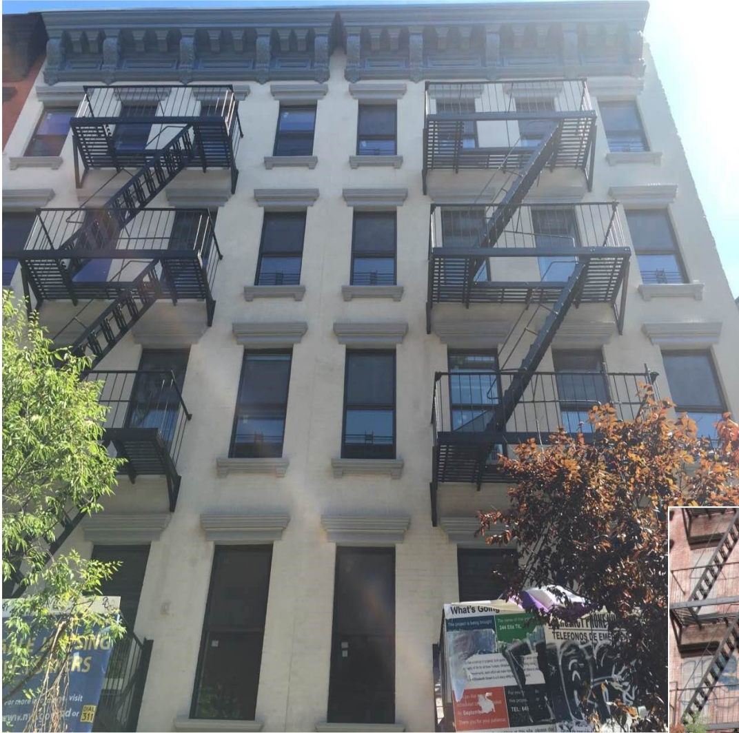
244 Elizabeth Post Renovation
