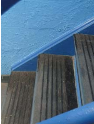
Fig. III-C-149 Stairwell A, Room 108, stair tread detail
