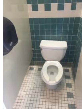
Fig. III-C-86 Room 212 Bathroom toilet stall
