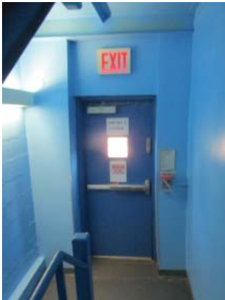
Fig. III-C-147 Stairwell A, Room 108, egress door to garden
