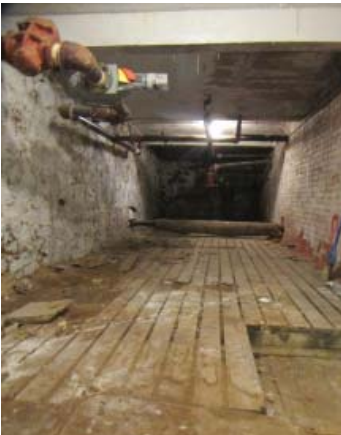
Fig. III-C-2 Room C01 Utilities Meter Room
