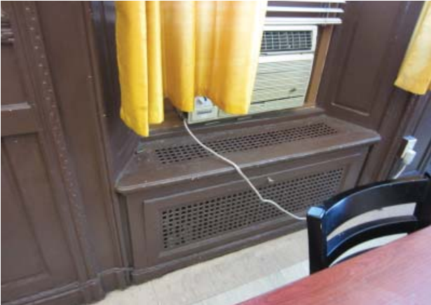
Fig. III-C-45 Room 106 Dining Room window vent
