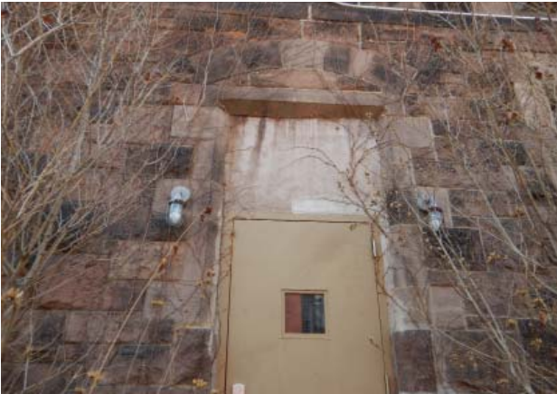
Fig. III-C-175 East Elevation Stairwell A door
