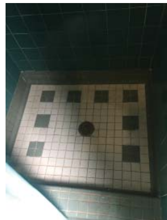
Fig. III-C-88 Room 212 Bathroom shower stall
