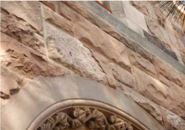
Fig. III-C-193 South Elevation detail of masonry deterioration
