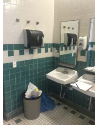
Fig. III-C-84 Room 212 Bathroom sinks
