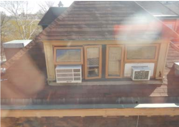
Fig. III-C-165 North Elevation detail
