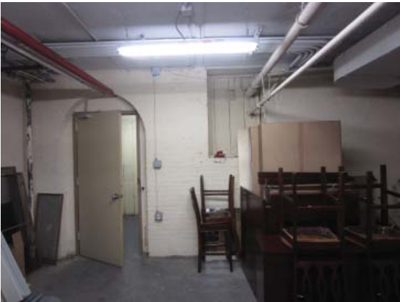
Fig. III-C-7 Room C02 Sprinkler Room
