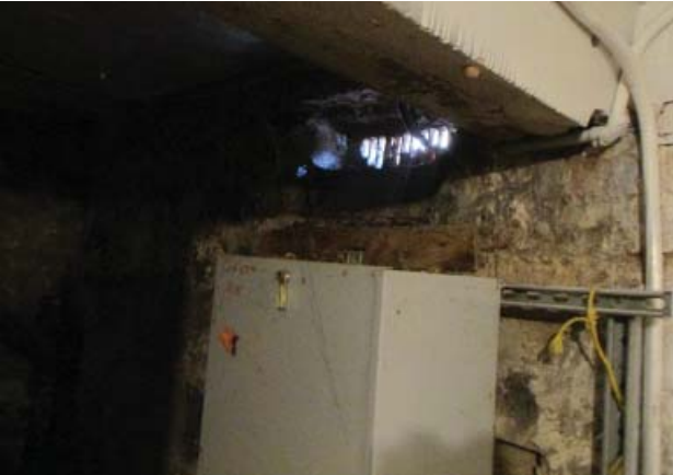
Fig. III-C-3 Room C01 Utilities Meter Room window
