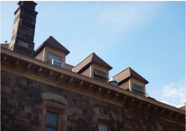
Fig. III-C-177 East Elevation detail of dormers
