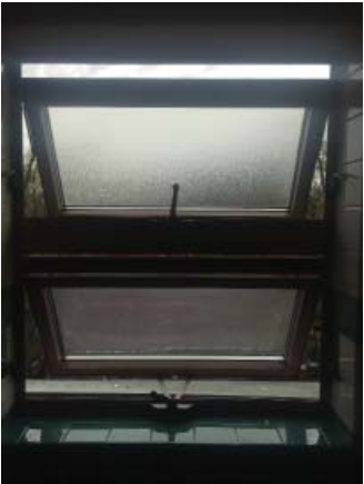
Fig. III-C-133 Room 306 Bathroom windows
