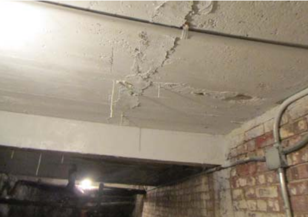
Fig. III-C-4 Room C01 Utilities Meter Room ceiling
