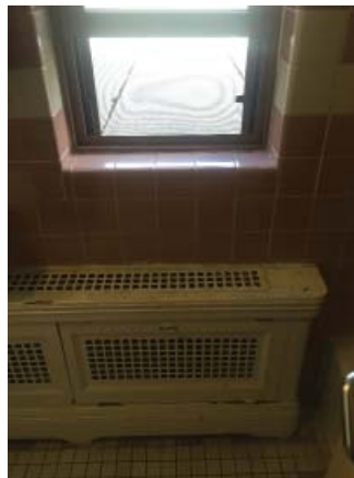
Fig. III-C-96 Room 216 Bathroom heater and window
