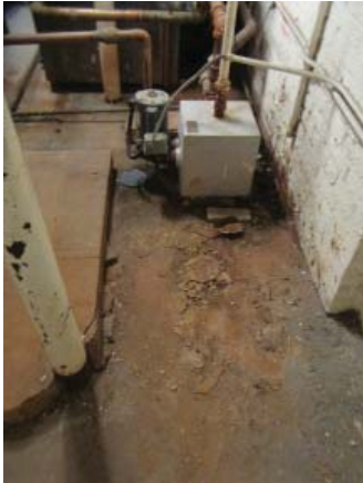
Fig. III-C-10 Room C03 Boiler Room
