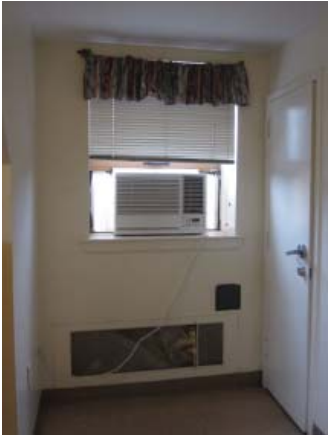
Fig. III-C-111 Room 301 Bedroom window
