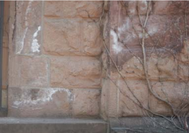
Fig. III-C-178 East Elevation detail of efflorescence
