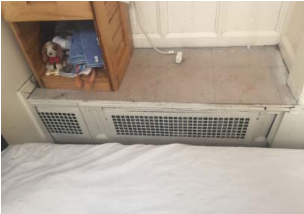
Fig. III-C-139 Room 308 Bedroom vent
