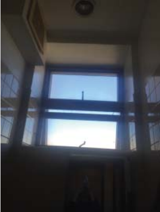
Fig. III-C-144 Room 310 Bathroom window
