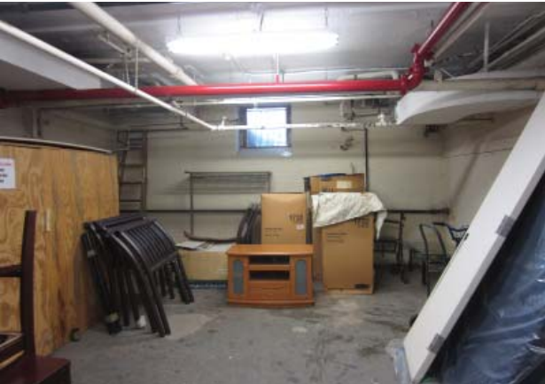
Fig. III-C-5 Room C02 Sprinkler Room
