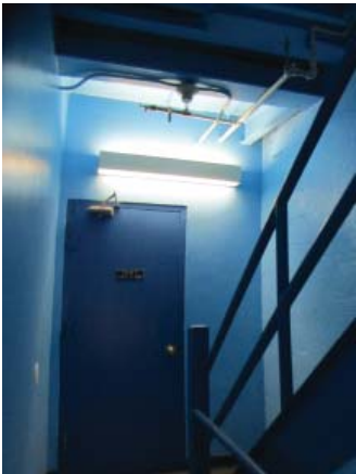
Fig. III-C-148 Stairwell A, Room 108, door to Room 105
