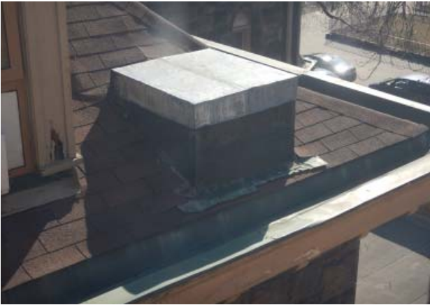
Fig. III-C-169 North Elevation detail
