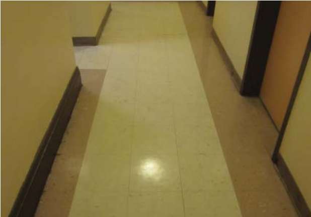
Fig. III-C-66 Room 205 Corridor floors
