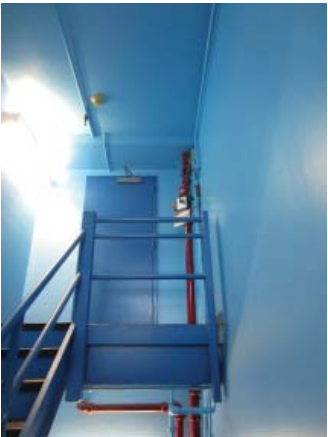
Fig. III-C-160 Stairwell B, Room 303, door to Room 305
