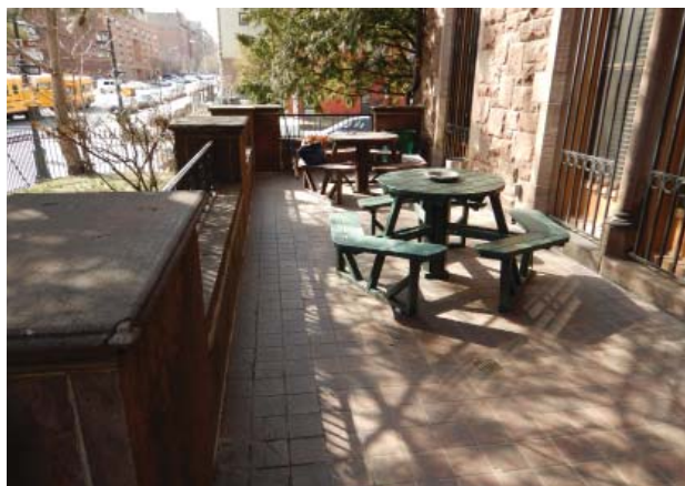
Fig. III-C-185 South Elevation front terrace
