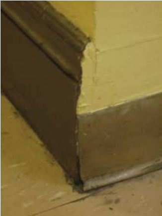
Fig. III-C-67 Room 205 Corridor baseboard
