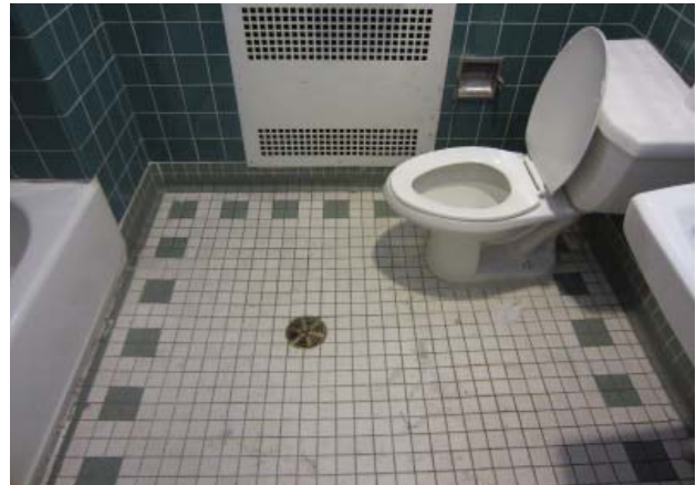
Fig. III-C-62 Room 204 Bathroom floor tiles
