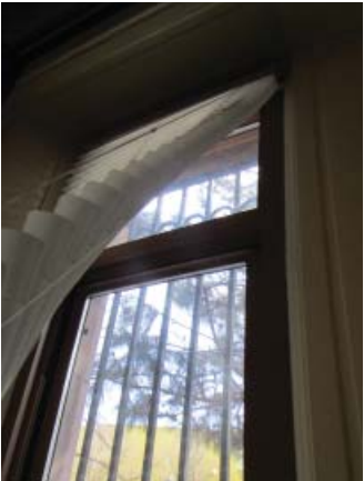
Fig. III-C-32 Room 101 Living Room window
