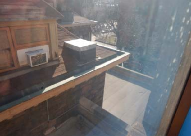
Fig. III-C-167 North Elevation detail
