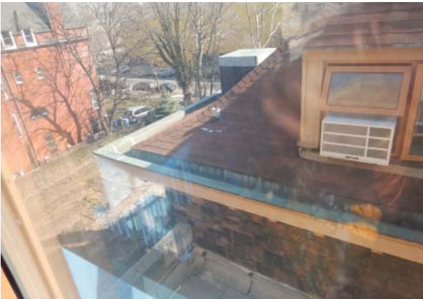
Fig. III-C-166 North Elevation detail
