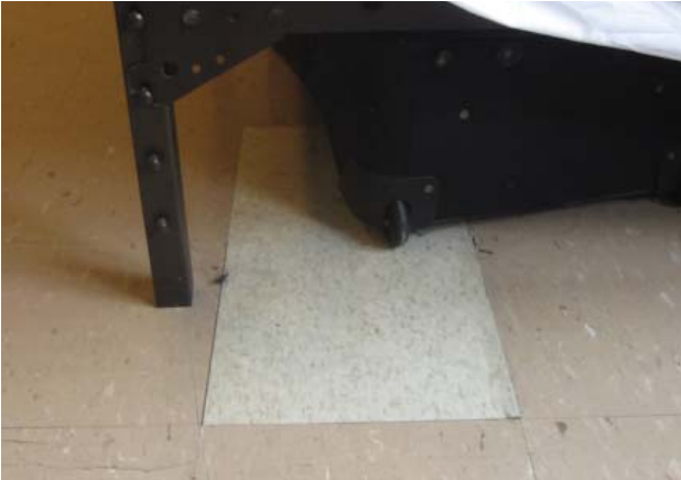
Fig. III-C-112 Room 301 Bedroom replacement floor tiles
