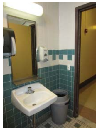
Fig. III-C-64 Room 204 Bathroom fixtures
