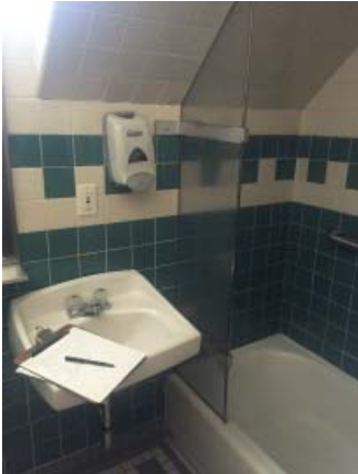
Fig. III-C-143 Room 310 Bathroom sink and tub
