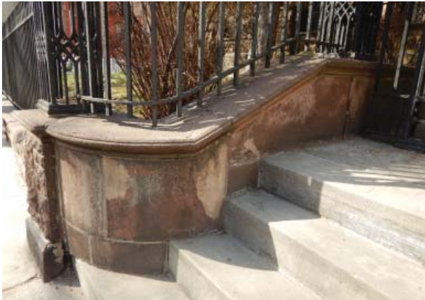
Fig. III-C-196 South Elevation detail of concrete steps and knee wall
