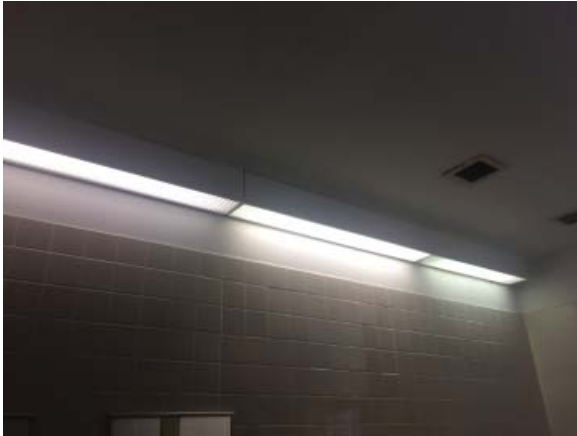
Fig. III-C-85 Room 212 Bathroom light fixtures
