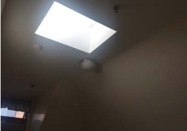
Fig. III-C-138 Room 308 Bedroom skylight
