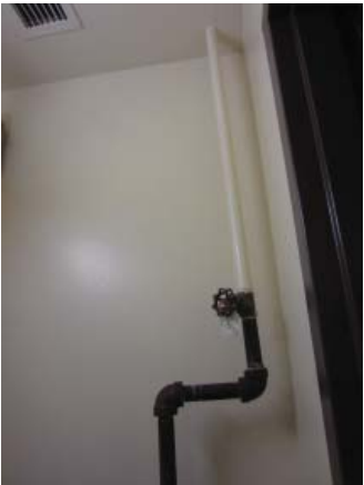
Fig. III-C-102 Room 217 Janitor's Closet pipe for utility sink
