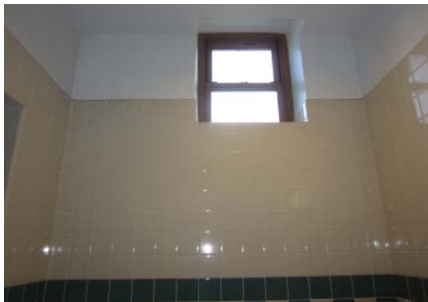
Fig. III-C-63 Room 204 Bathroom upper wall and window
