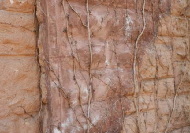
Fig. III-C-179 East Elevation detail of trapped moisture, III-Cne growth and efflorescence
