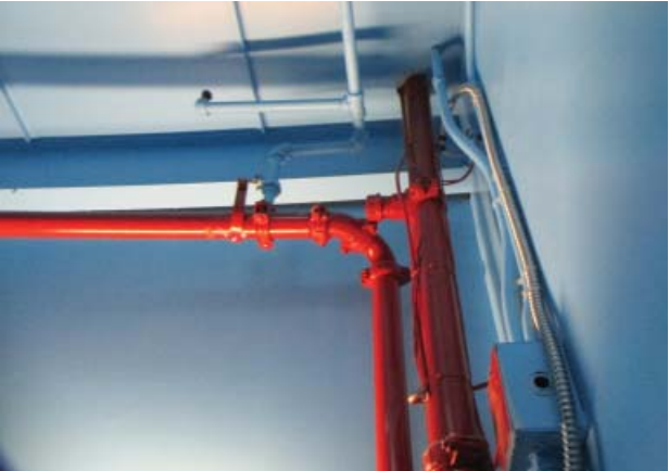
Fig. III-C-156 Stairwell B, Room 103 pipes
