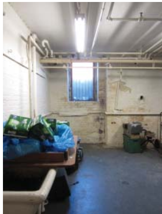
Fig. III-C-23 Room C09 Storage Room
