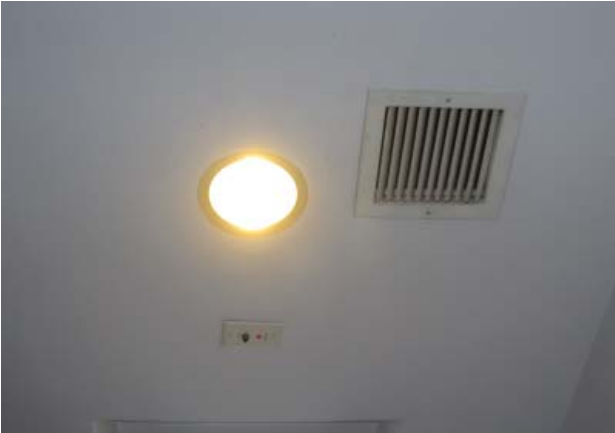
Fig. III-C-65 Room 204 Bathroom ceiling light and vent
