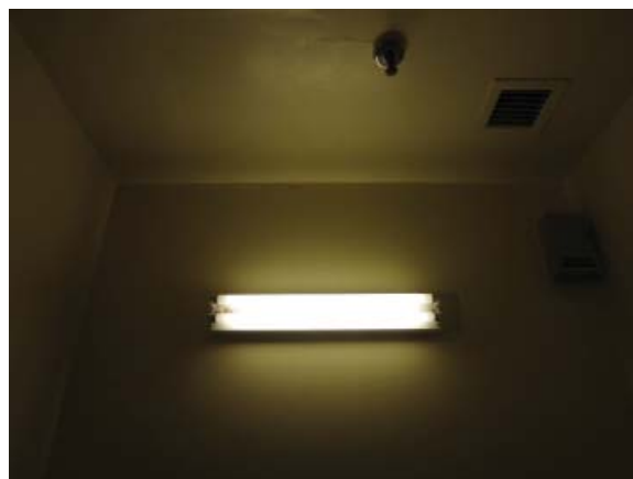
Fig. III-C-100 Room 217 Janitor's Closet ceiling and light fixture
