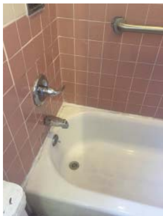
Fig. III-C-97 Room 216 Bathroom tub
