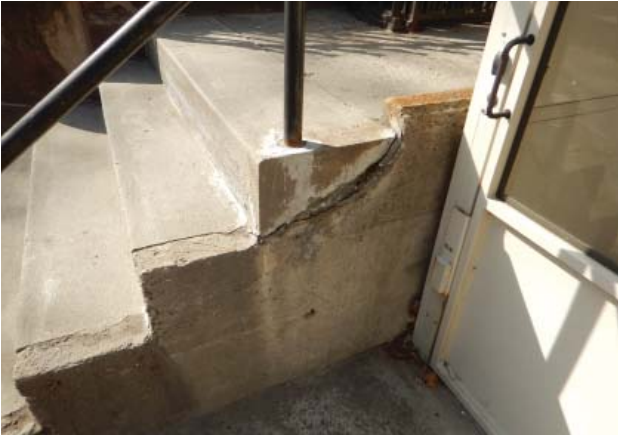
Fig. III-C-189 South Elevation detail of entry steps
