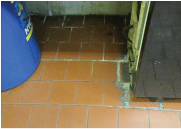
Fig. III-C-51 Room 109 Kitchen floor tiles
