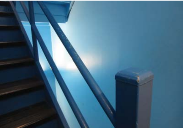
Fig. III-C-158 Stairwell B, Room 209, paint peeling on railing
