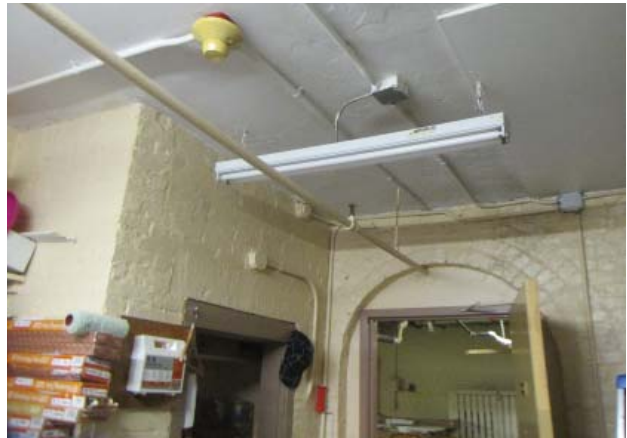
Fig. III-C-22 Room C08 Storage Room ceiling
