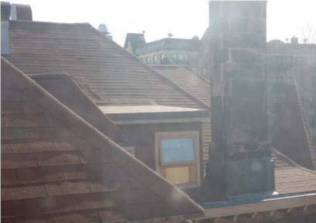
Fig. III-C-168 North Elevation detail
