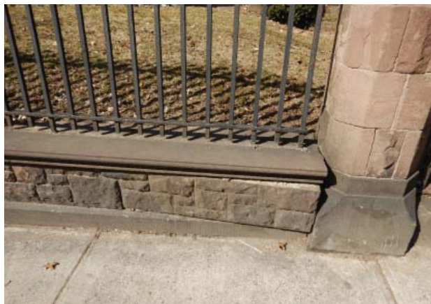
Fig. III-C-187 South Elevation displacement at fence knee wall and newels
