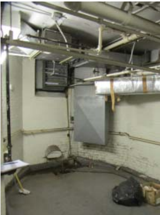
Fig. III-C-8 Room C03 Boiler Room
