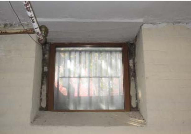
Fig. III-C-6 Room C02 Sprinkler Room window
