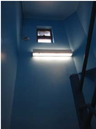
Fig. III-C-159 Stairwell B, Room 303, window
