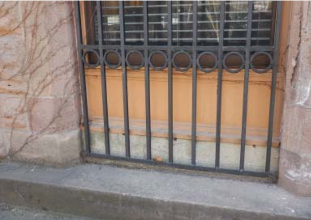
Fig. III-C-172 East Elevation window on one story front projection
