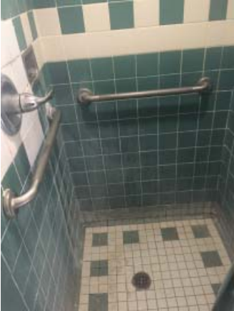
Fig. III-C-132 Room 306 Bathroom shower
