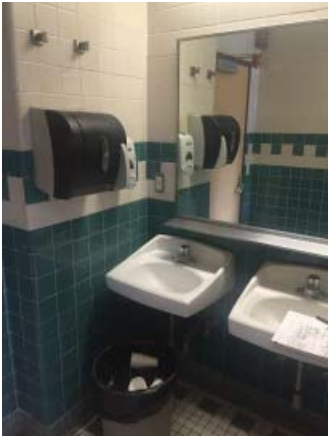
Fig. III-C-127 Room 306 Bathroom sinks
