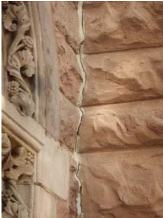
Fig. III-C-194 South Elevation detail of large scale crack between facade plane and one story projecting addition
