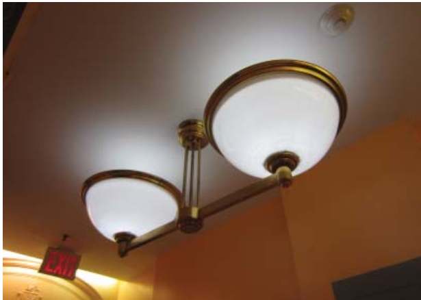
Fig. III-C-41 Room 105 Corridor light fixture
