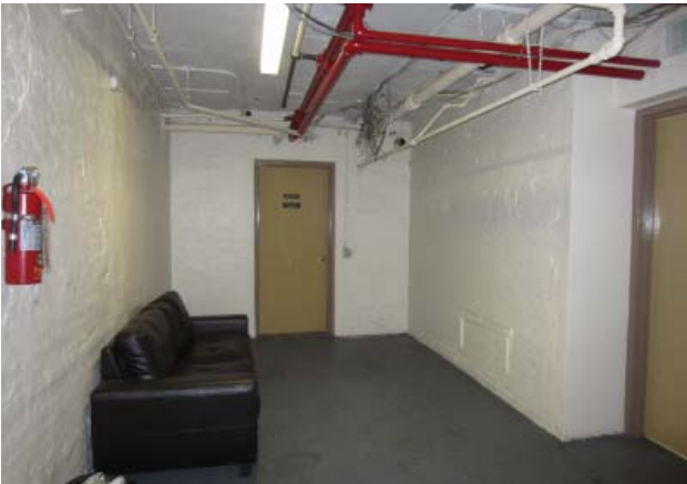
Fig. III-C-14 Room C05 Corridor
