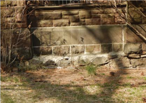
Fig. III-C-191 South Elevation water table detail
