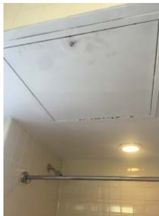
Fig. III-C-98 Room 216 Bathroom ceiling
