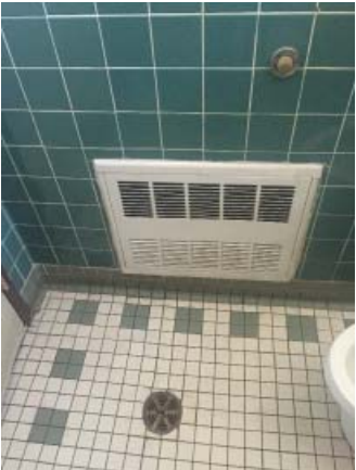
Fig. III-C-146 Room 310 Bathroom vent
