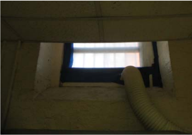
Fig. III-C-18 Room C06 Chart Room window
