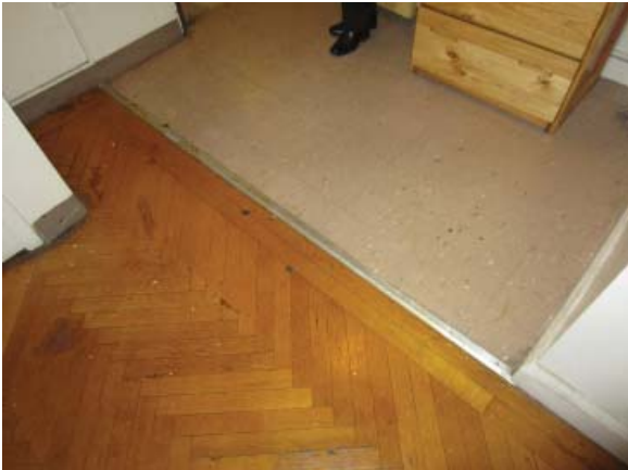
Fig. III-C-69 Room 206 Bedroom floors
