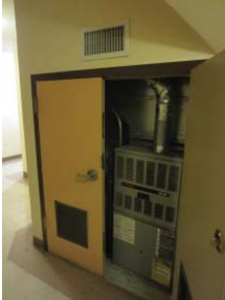
Fig. III-C-126 Room 305 Corridor mechanical room
