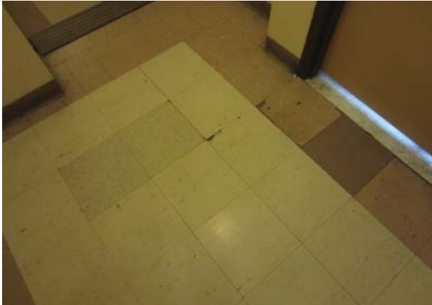
Fig. III-C-125 Room 305 Corridor areas of replacement tiles
