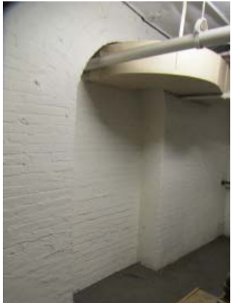
Fig. III-C-11 Room C03 Boiler Room arched opening infilled with brick
