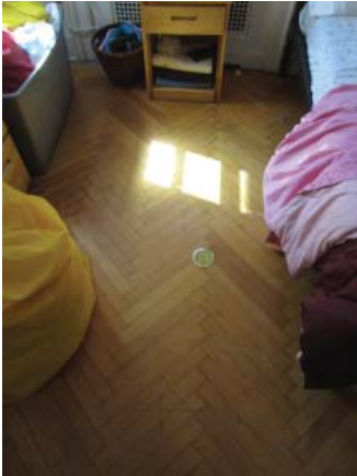
Fig. III-C-54 Room 201 Bedroom wooden floor laid in herringbone pattern
