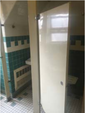
Fig. III-C-131 Room 306 Bathroom stalls
