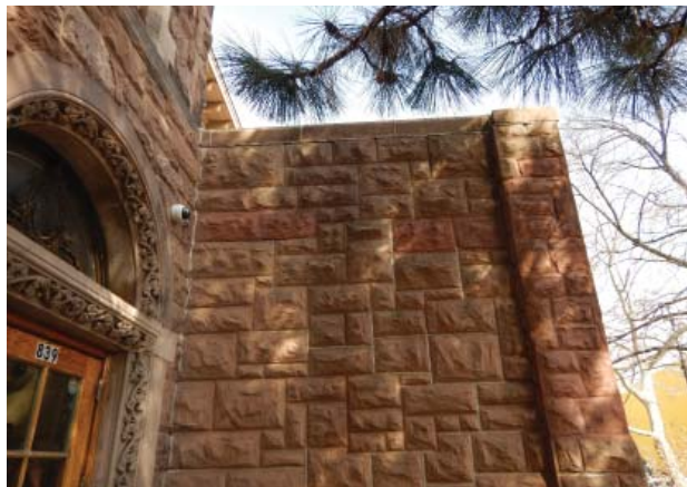
Fig. III-C-183 South Elevation crack between facade plane and one story projecting addition
