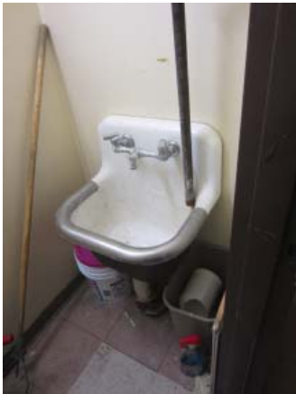
Fig. III-C-101 Room 217 Janitor's Closet utility sink
