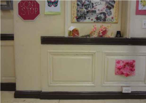
Fig. III-C-36 Room 102 Library wainscoting
