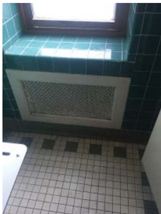
Fig. III-C-87 Room 212 Bathroom vent
