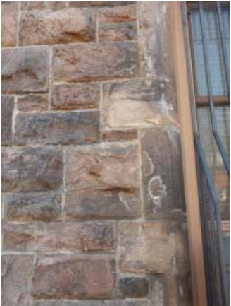
Fig. III-C-180 East Elevation detail of spalling masonry
