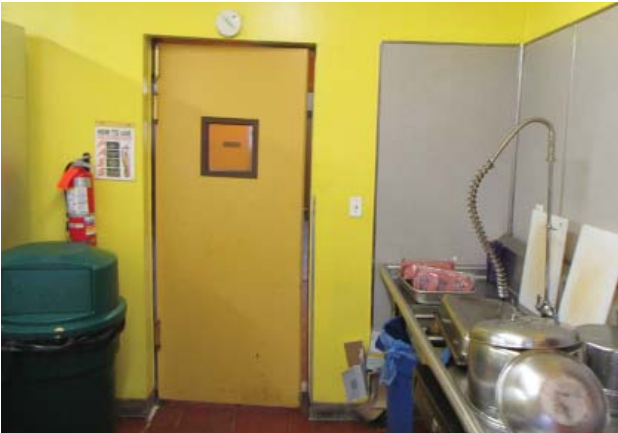
Fig. III-C-50 Room 109 Kitchen door
