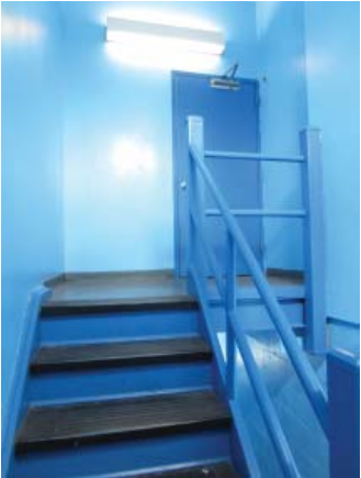
Fig. III-C-154 Stairwell A, Room 307, door to Room 305
