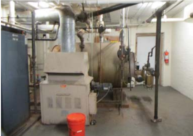
Fig. III-C-9 Room C03 Boiler Room
