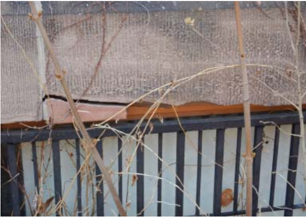
Fig. III-C-174 East Elevation window detail of Room C08
