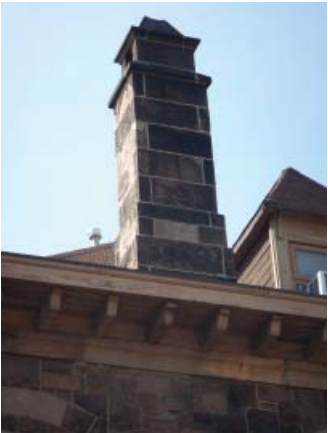
Fig. III-C-181 East Elevation detail of chimney
