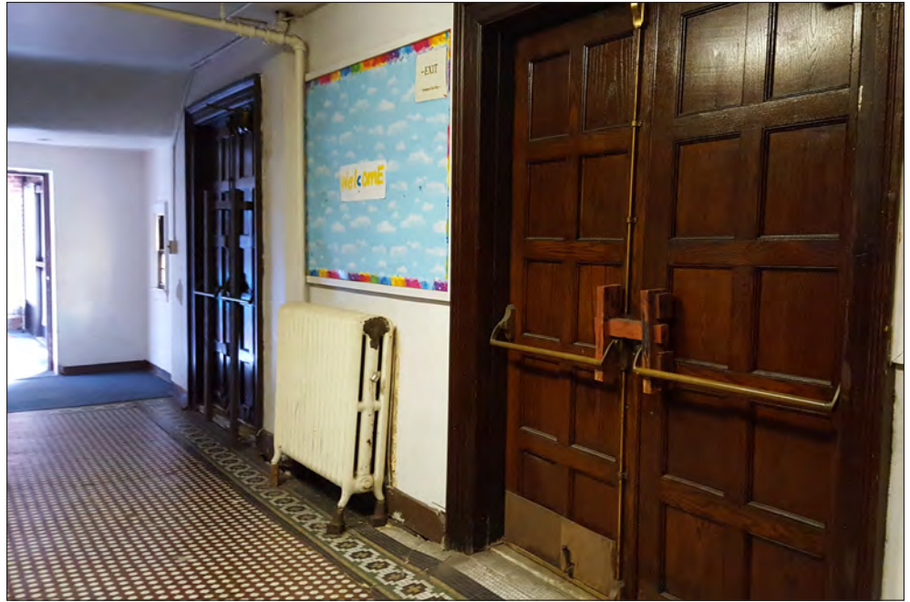
View south in the ground floor lobby/hallway towards the one-story connector structure that links to the educational building. 5
