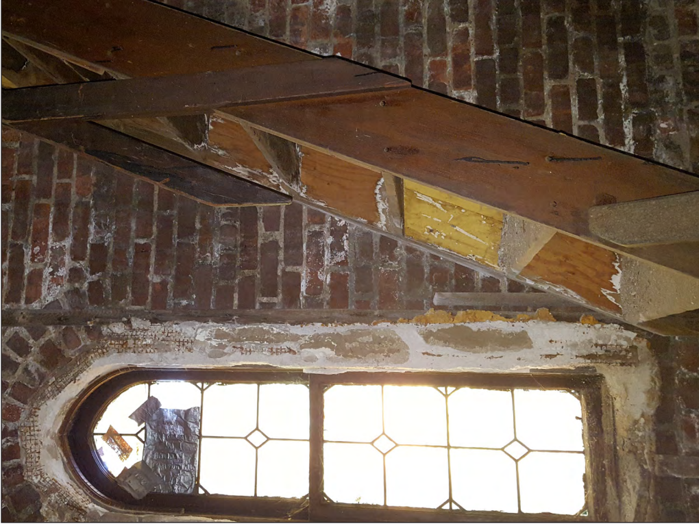
View of ladder leading to formerly open belfry in the church tower. 14
