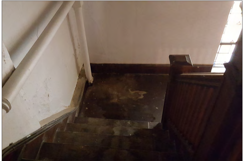
View looking down from stair landing at balcony level, towards stained glass window on the north façade of the church at the north stair landing. 15
