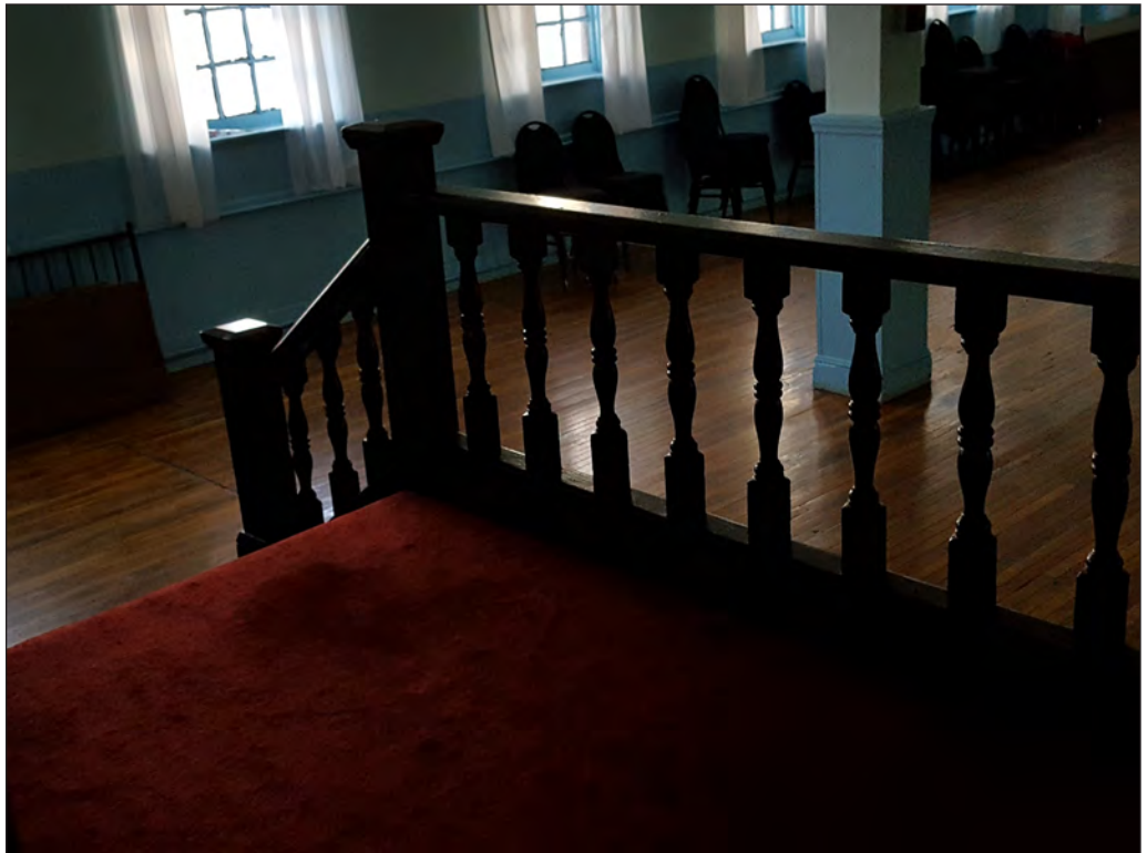
View of one of the stairs from the landing that provide access from the ground floor hallway level to the basement level multi-purpose room. 4
