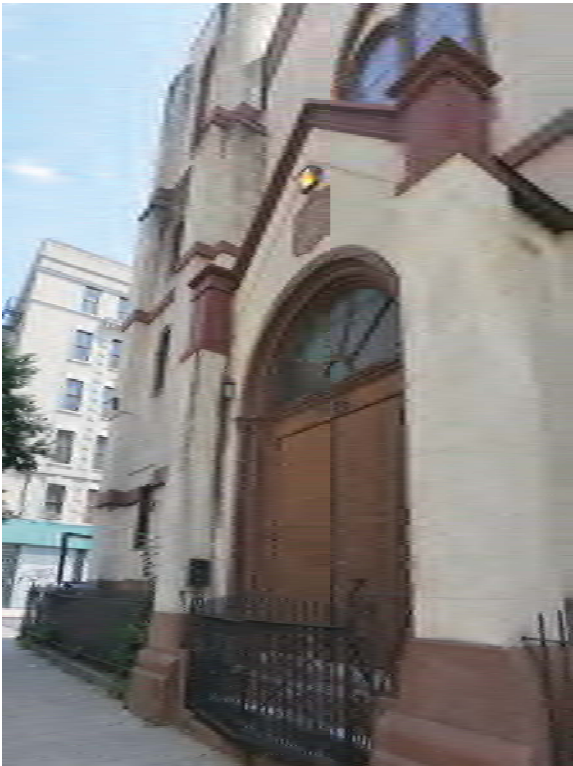
Photo 2: View north of the Church's entrance on Washington Avenue.
