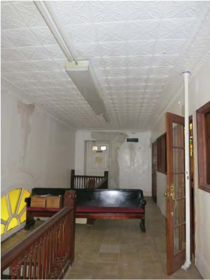
Photo 10: View north in the second floor lobby/hallway of the church. A bathroom, installed in 1937 is at the end of the hall.
