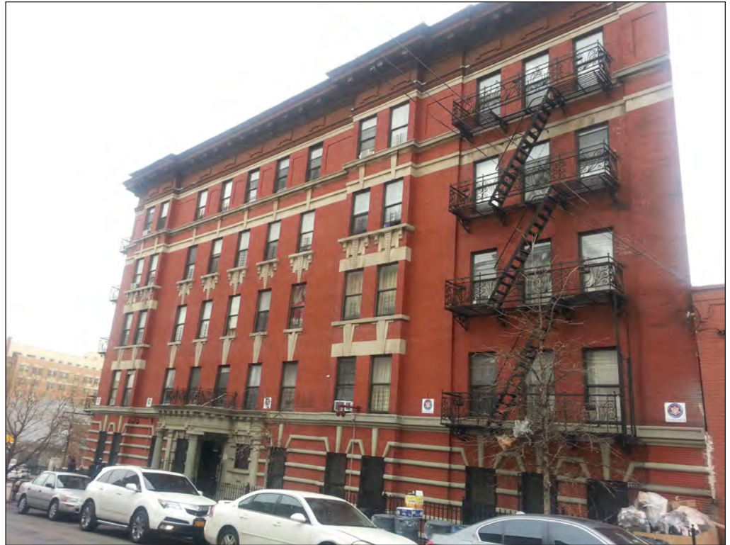
View southwest of the Franklin Avenue façade of the Franklin Court Apartments at 1071 Franklin Avenue 3
