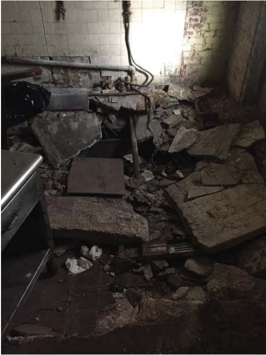
Photo 12b: collapsed floor in the former kitchen on the first floor.
