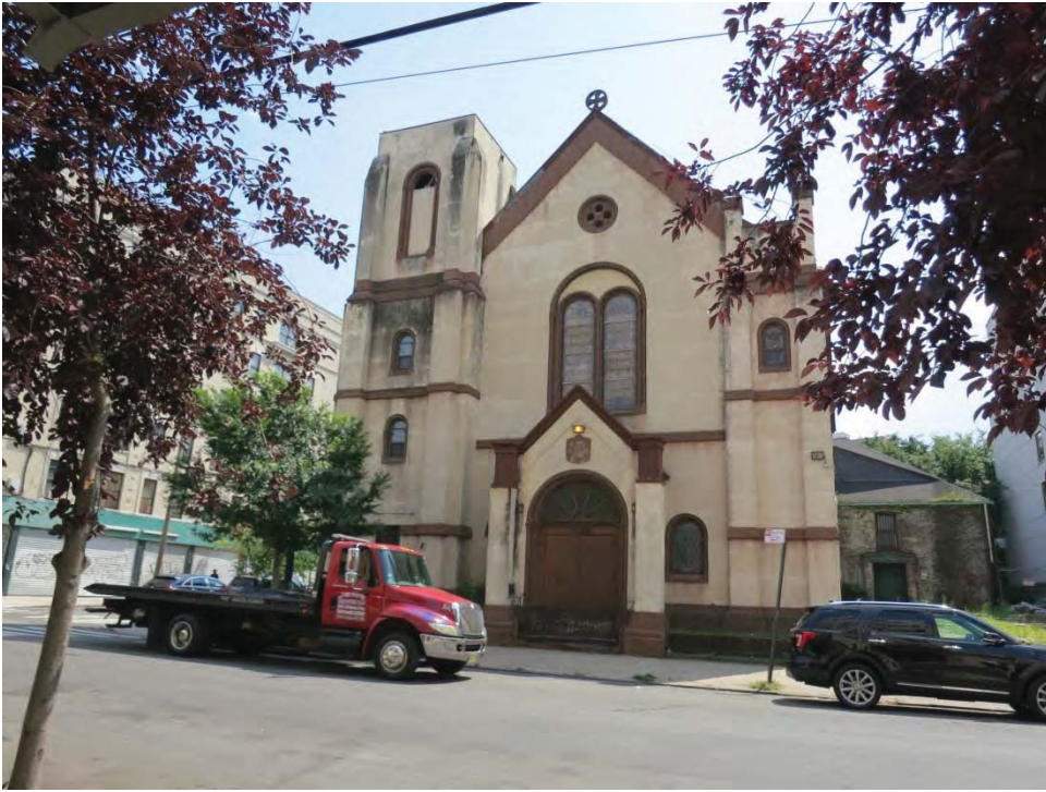
Photo 1: View east of Washington Avenue (principal façade) of the former Centenary Methodist Episcopal Church.
