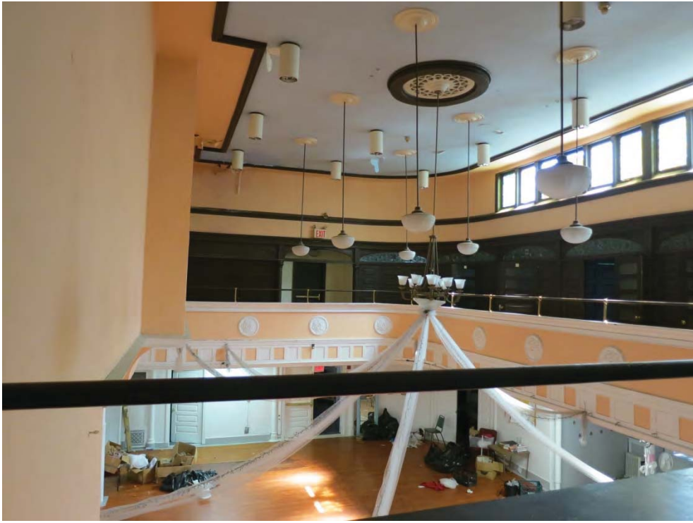
Photo 21: View north at the balcony level in the Sunday School building.
