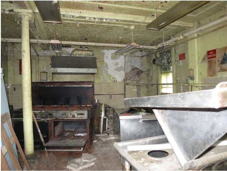
Photo 12a: Former kitchen on the first floor of the Church along East 166th Street.
