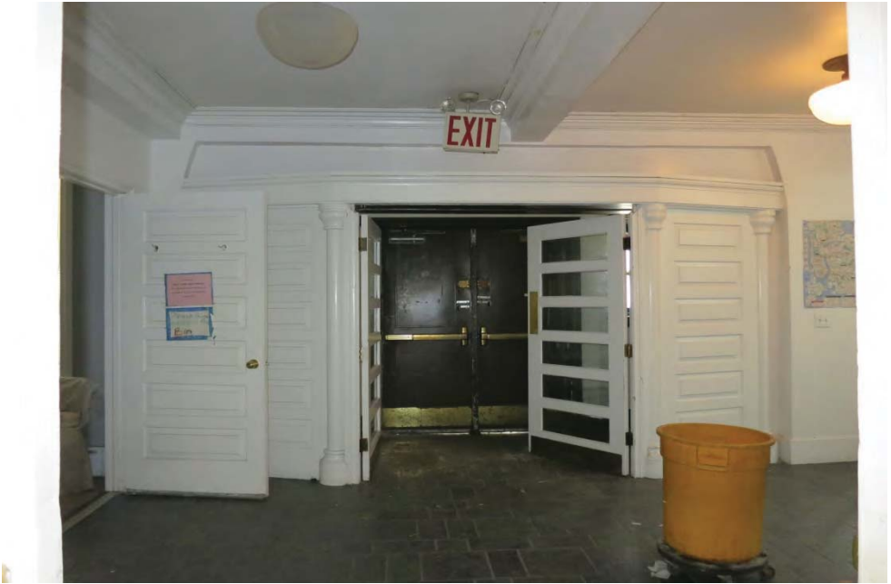
Photo 18: View of the entrance to East 166th Street in the Sunday School first floor lobby.
