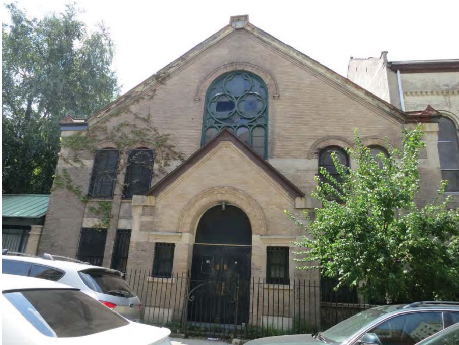
Photo 4: View of the 1902/1903 Sunday School building on East 166th Street.
