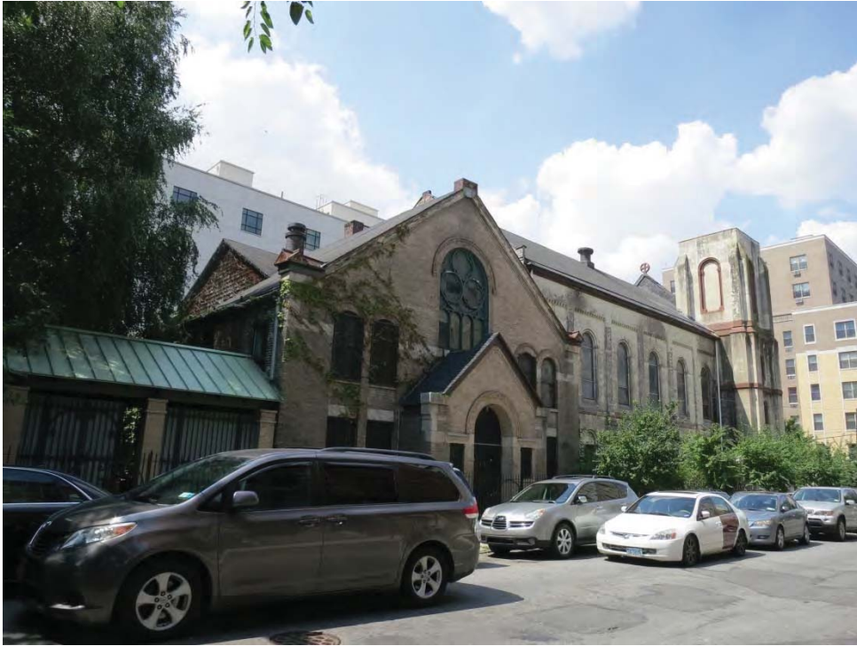
Photo 3: View southwest on East 166th Street of the Centenary Methodist Episcopal Church. The 1902/1903 Sunday School building is on the left with the main church structure on the right. A more recent one-story addition is on the far left.
