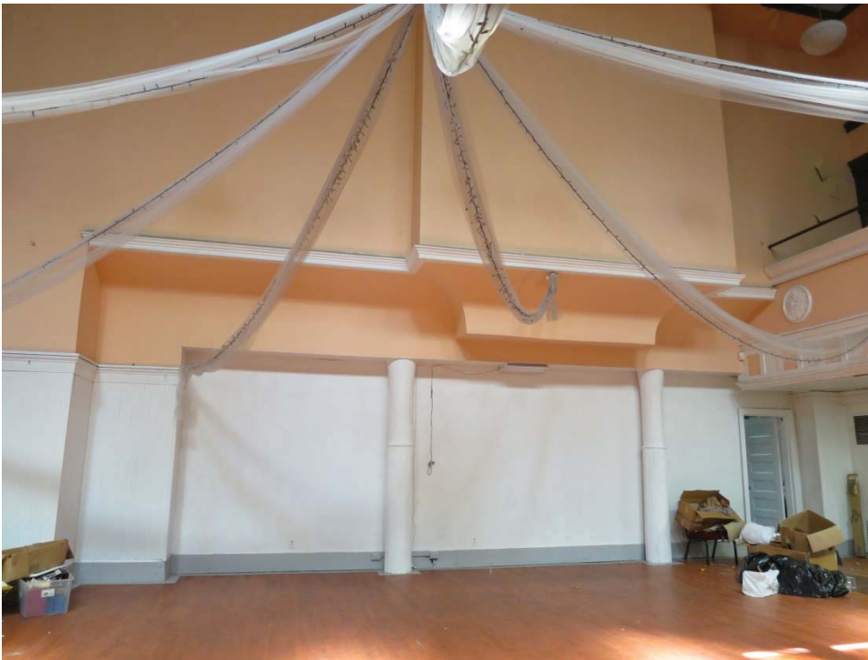
Photo 20: View west towards the connecting wall between the church and the Sunday School building. The doorway at the right provides access to the church's modernized first floor space.
