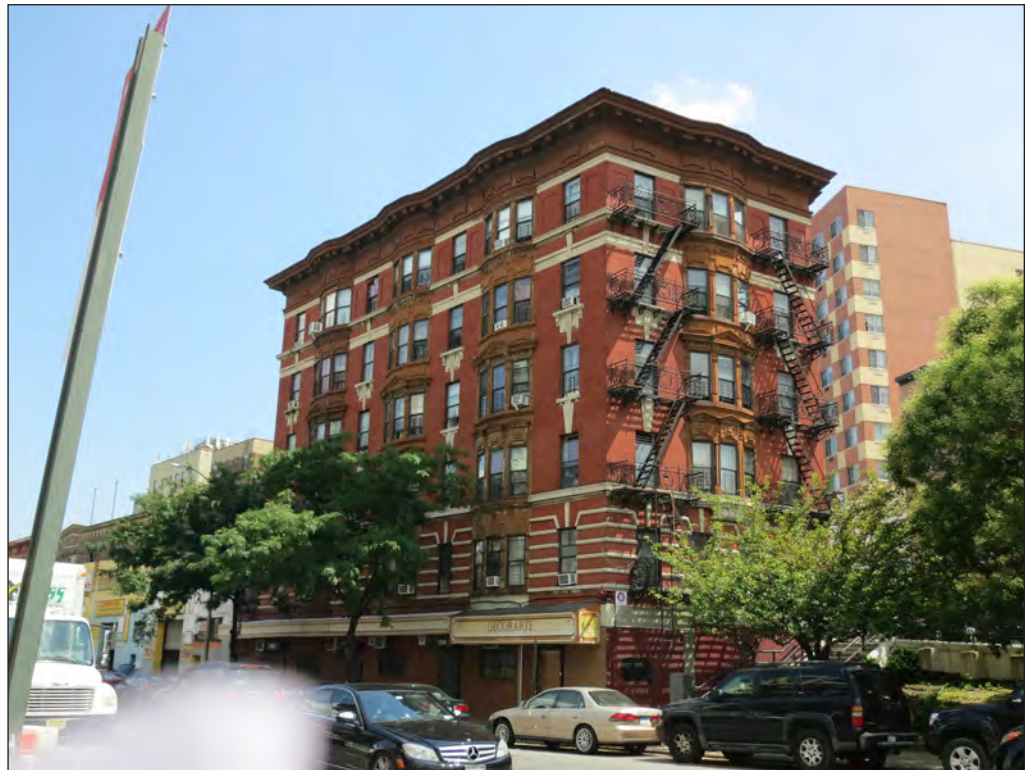
View northeast of the west (Third Avenue) and south façades of the Franklin Court Apartments 4
