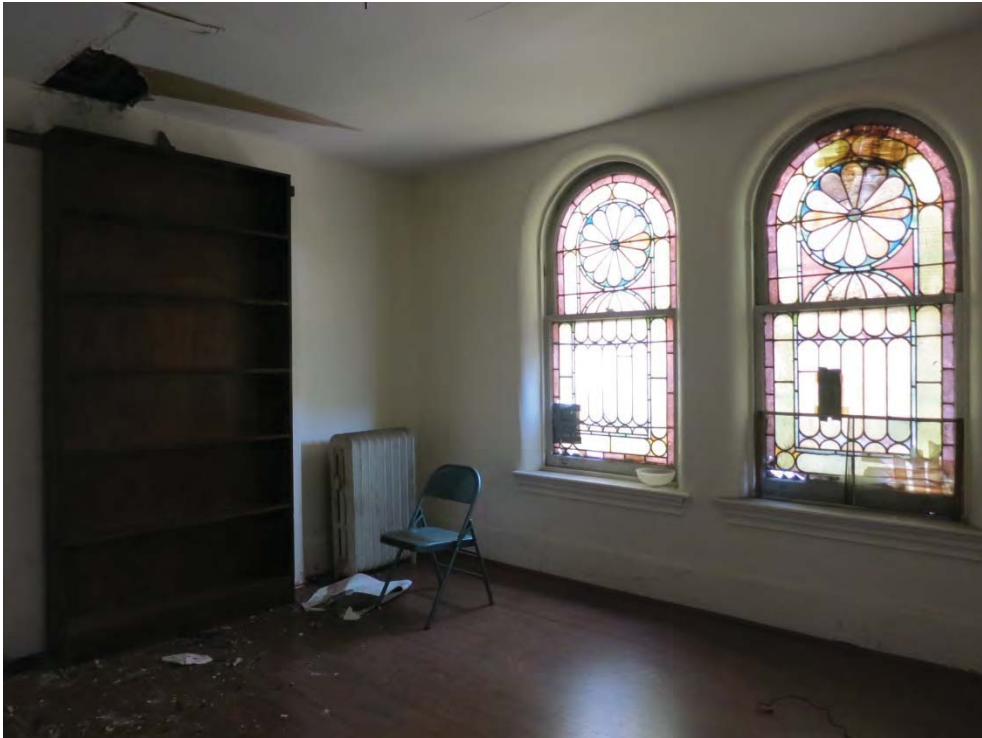
Photo 22: Room in the Sunday School adjacent to the Church; the stained glass windows (broken) front onto East 166th Street).
