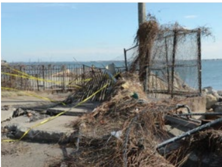
Damage to the Coney Island waterfront.
