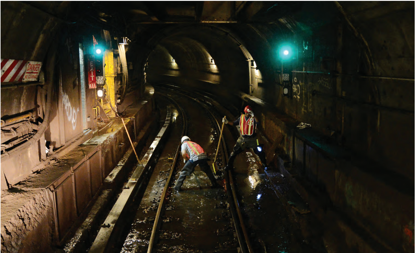
Cortlandt Street Tunnel (Photo Credit: © Metropolitan Transit Authority / Marc A. Hermann)
