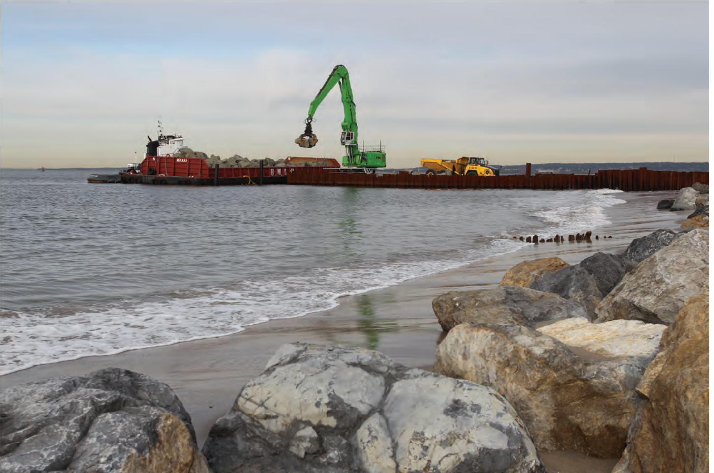
Construction of coastal protection at Sea Gate in Brooklyn.
