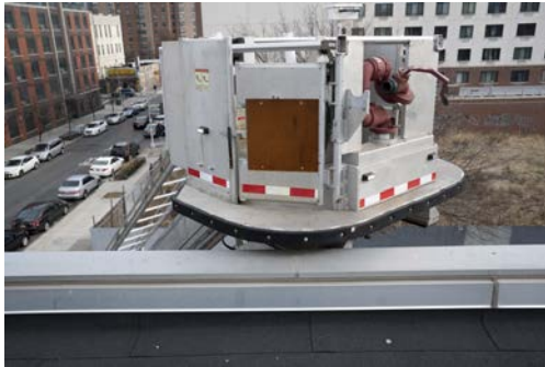
Photo 4 - Bucket Placed to Roof
