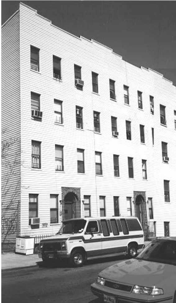
OLD LAW TENEMENT TYPE ROW FRAME BUILDINGS WITH A FOUR-WINDOW FRONT (Refer to Text Section 5.1.2 B)
