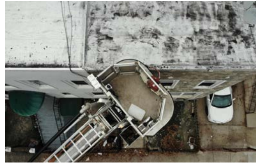
Photo 5 - Bucket Placed to Roof
