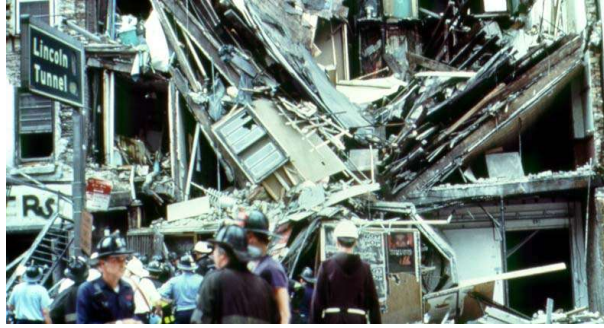
Figure 5: V-shaped collapses produce large voids along the remaining walls. These voids are likely locations to find survivors.
