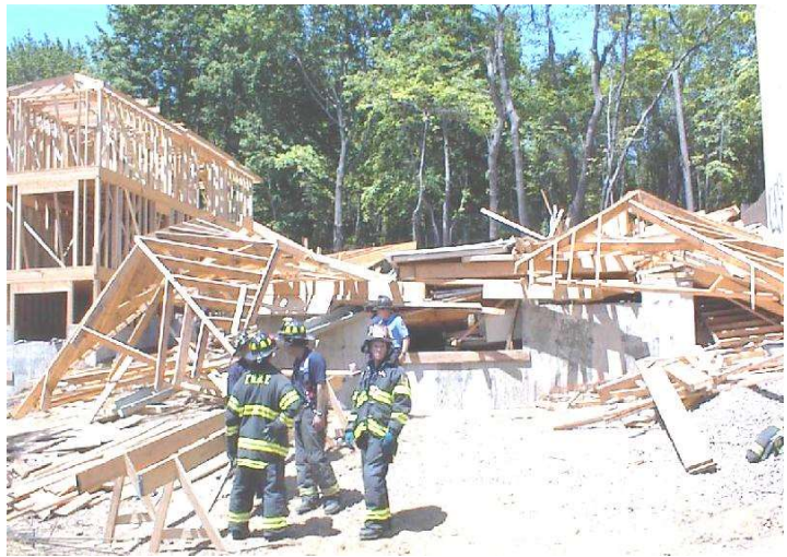
Figure 6: This two-story frame home under construction pancaked straight down, trapping one worker in the basement. The worker was face down in wet concrete. The floors above were prevented from reaching the lowest floor by the foundation walls that created a void one-to-two feet high in the basement.
