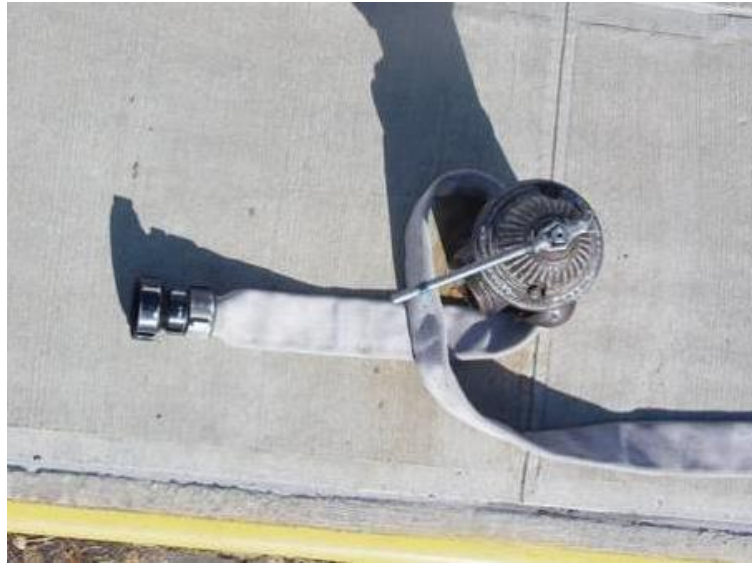
Hydrant keyed with 3 ½" hose:
