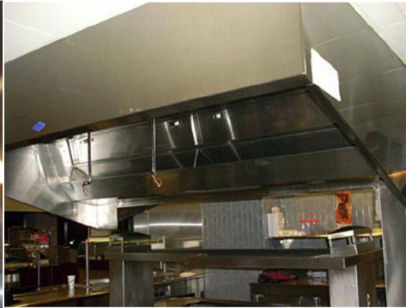
TYPE I HOOD WASH HAS PLENUM DOORS
