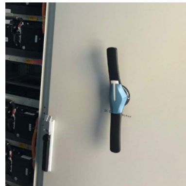
Battery container disconnect switch
