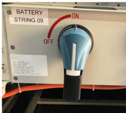
Battery string disconnect switch
