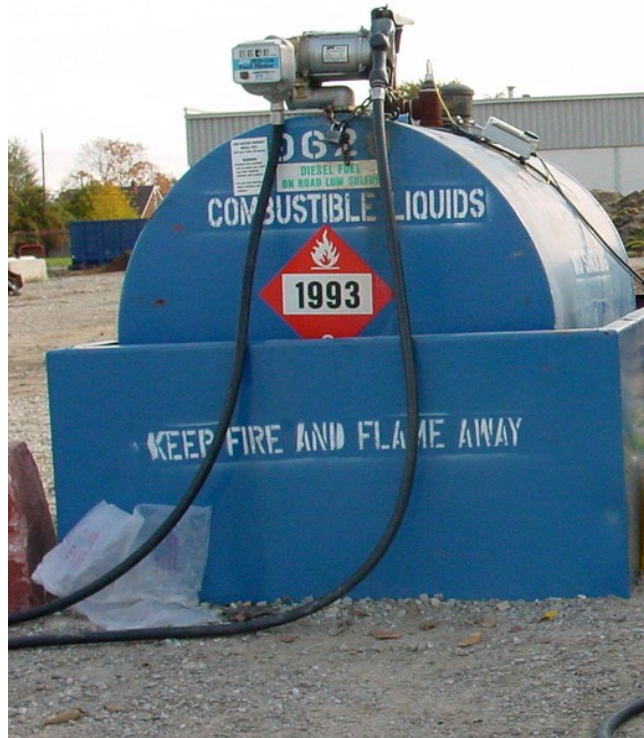
Example of a temporary tank with top openings.
