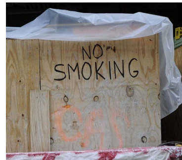
Unacceptable Warning Sign
