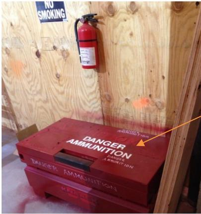
The ammunition storage box must be locked and properly labeled.
