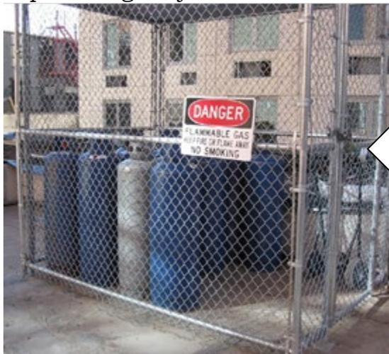
The propane cylinders must be stored in a well-ventilated outdoor enclosure secured by a lock. They must not be stored in any below grade area.
