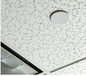
A photograph showing a concealed sprinkler head installed in a ceiling. The head is a white, circular plate flush with the surface of a white, textured acoustic ceiling tile. The surrounding ceiling is made of similar tiles, and a portion of a white ceiling grid is visible at the bottom. |
