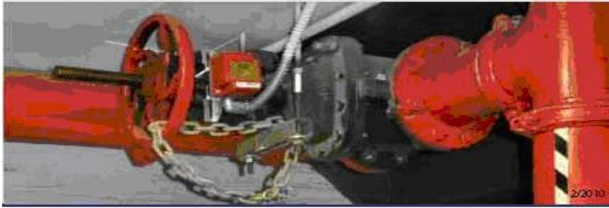
**TESTING** - A procedure used to determine the status of a system as intended by conducting periodic physical checks on water based fire protection systems such as water-flow tests, fire pump tests, alarm tests, and trip tests of dry pipe, deluge, or preaction valves. These tests follow up on the original acceptance test at intervals specified in the appropriate chapter of NFPA #25, 2011 edition.
