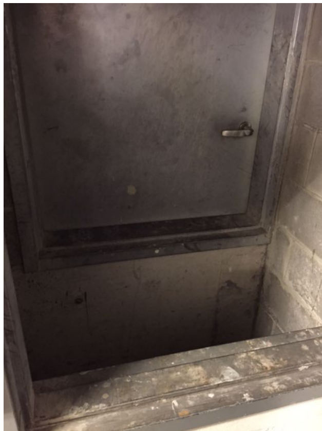
MAIN OIL STORAGE TANK DIKE
