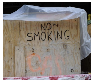
Unacceptable Warning Sign
