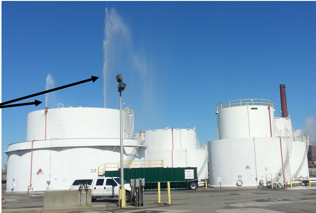
PART OF A 2-YEAR FOAM CONCENTRATE TEST
