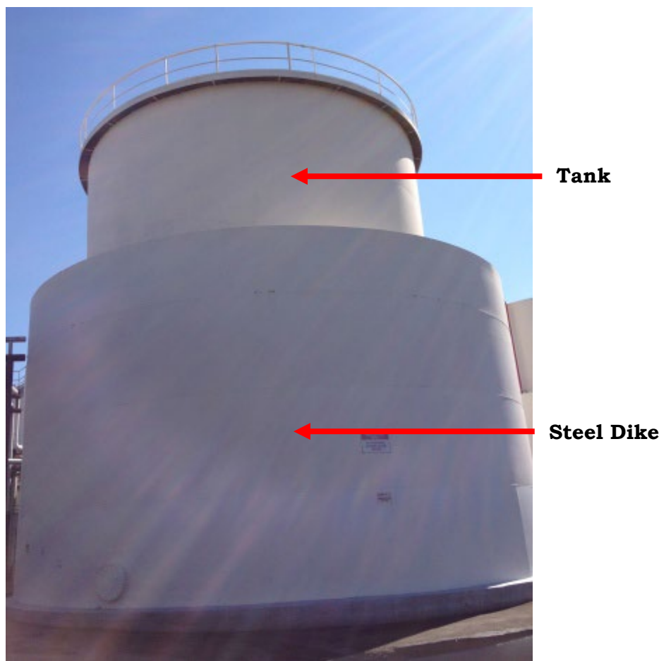
Above Ground Tank and Dike
