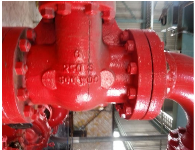
Damaged Valves
