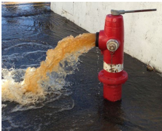
Testing a hydrant (part of a two-year test)
