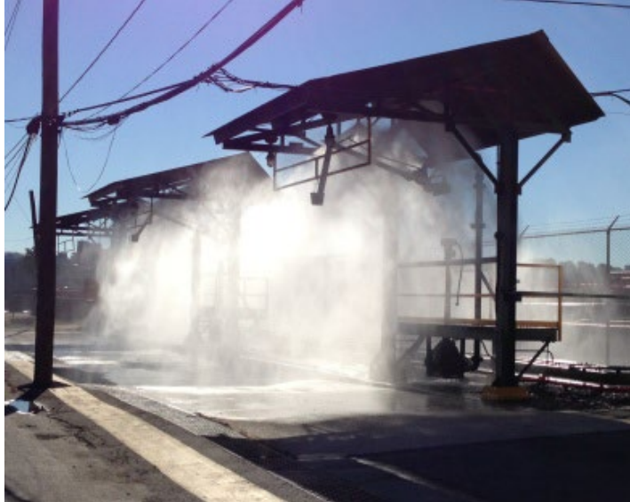
Fog Sprinkler System (activated)
