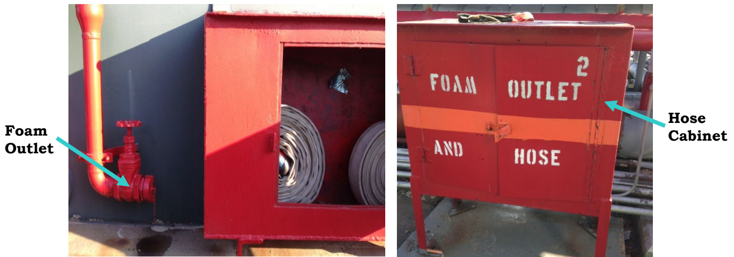
(L) Hose Cabinet and Foam Outlet. (R) Foam Outlet
