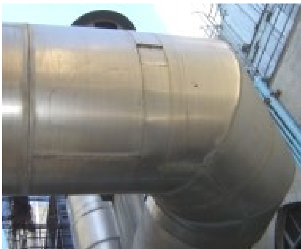
Exhaust Duct at a Co-Generation Plant
