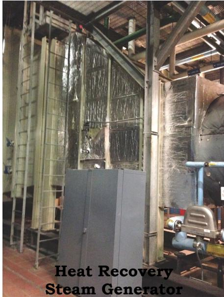
The **breeching and stack** is a channel, vertical pipe, chimney, or similar structure through which combustion product gases called flue gases are exhausted to the atmosphere. It may consist of pipes throughout a building system until it directs the flue gases to a proper place to be released. Flue gases are produced when natural gas or any other fuel is combusted in a HRSG, boiler, turbine, or engine.
