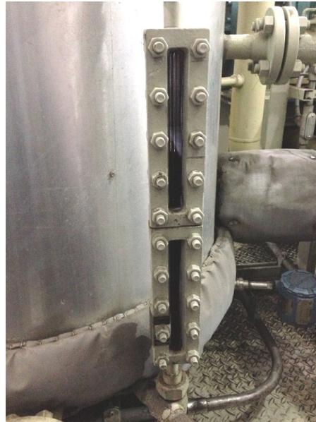
**Monitoring Oil Level in Separator Tank**
