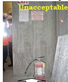
Improper floor placement of Fire Extinguisher.
