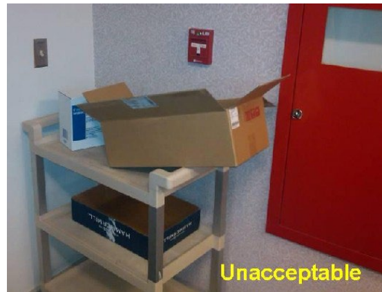
Obstructed Manual Pull Station
