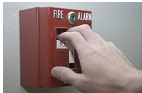
Activate a single action station
