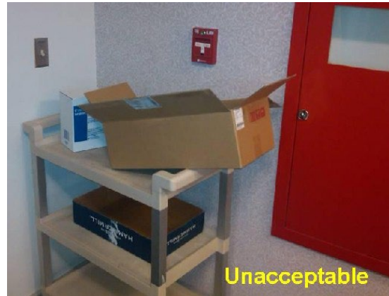
Obstructed Manual Pull Station
