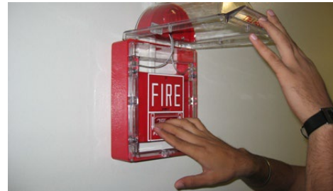
Activate a double action station
