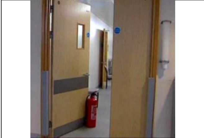
Fire doors propped open using a portable fire extinguisher ( illegal )
