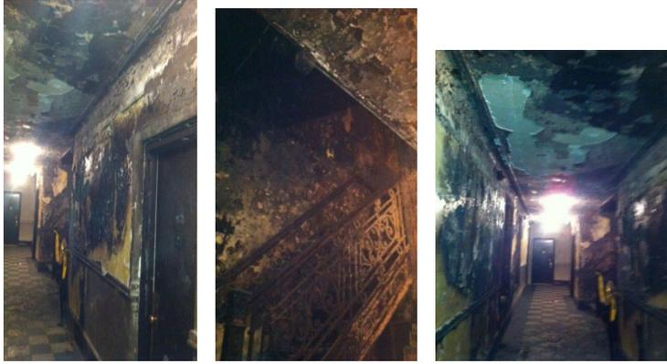
Pictures show the interior of the Bronx, NY shelter after the second mattress fire. There was severe smoke and fire damage in the hallways and stairwells.
