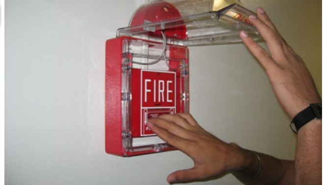
Activate a double action station
