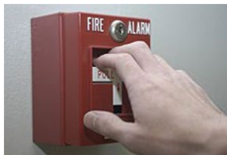
Activating a single action station
