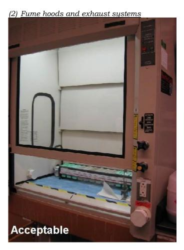
Approved fume hoods and exhaust systems which are installed to limit work place exposure to hazardous or noxious fumes, vapors or dusts. In general, fresh air is drawn in from the open side of the fume hood, and expelled outside the building (ducted type fume hood). Although commonly used outside N.Y.C., hoods made safe through filtration and fed back into the room are not allowed to be used in the city.
