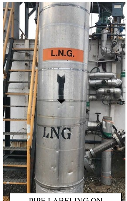
PIPE LABELING ON VAPORIZER
