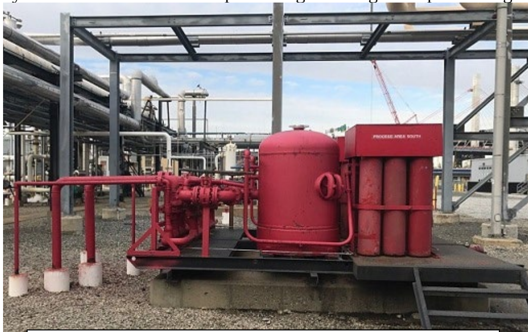
DRY POWDER UNIT WITH ISOLATING VALVES
