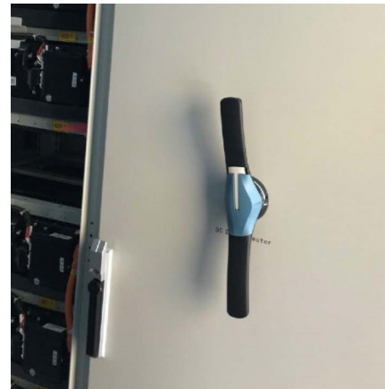
Battery container disconnect switch
