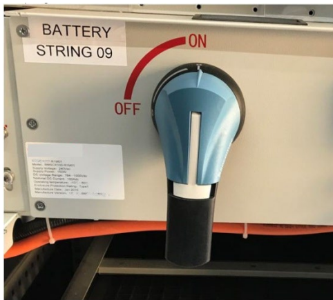
Battery string disconnect switch
