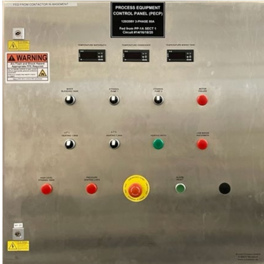
Electrical: Temperature control readings for different parts of still.
