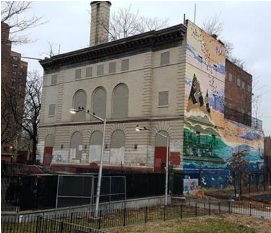
South & East Facade
