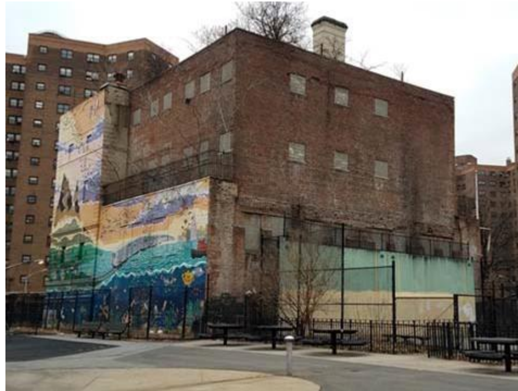
North & East Facade
