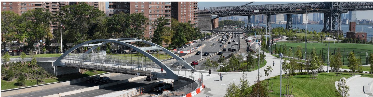
Park access via Corlears Hook bridge, September 2025
