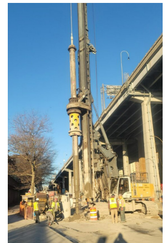
Sewer installation on Lewis Street (left) and secant pile installation on Delancey Street S (right), December 2025
