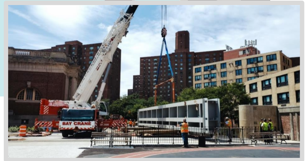
Floodgate 18 installed at Asser Levy Playground
