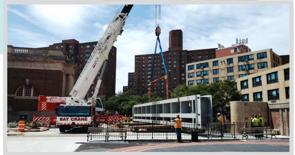
Floodgate 18 installed at Asser Levy Playground
