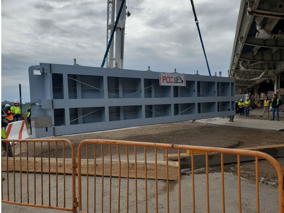
Stuyvesant Cove Park Vehicular Swing Gate install 2/24/2022
