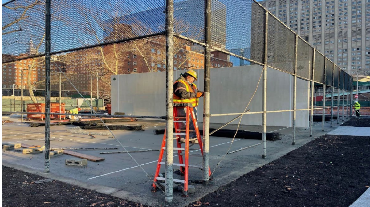
Asser Levy Playground handball court reconstruction
