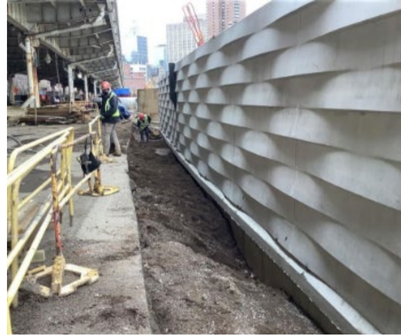
Stuyvesant Cove Park floodwall (looking north)
