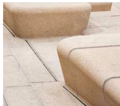
PRECAST CONCRETE SEATWALLS
