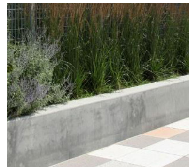
C.I.P. CONCRETE SITE WALLS
