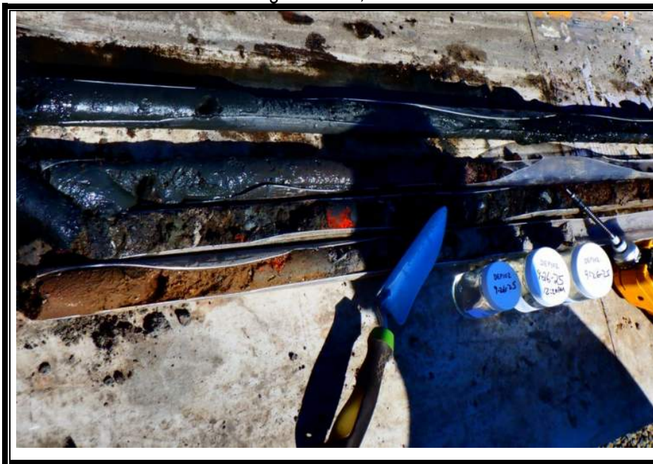
Soil boring DEP-102, collected 9/26/25
