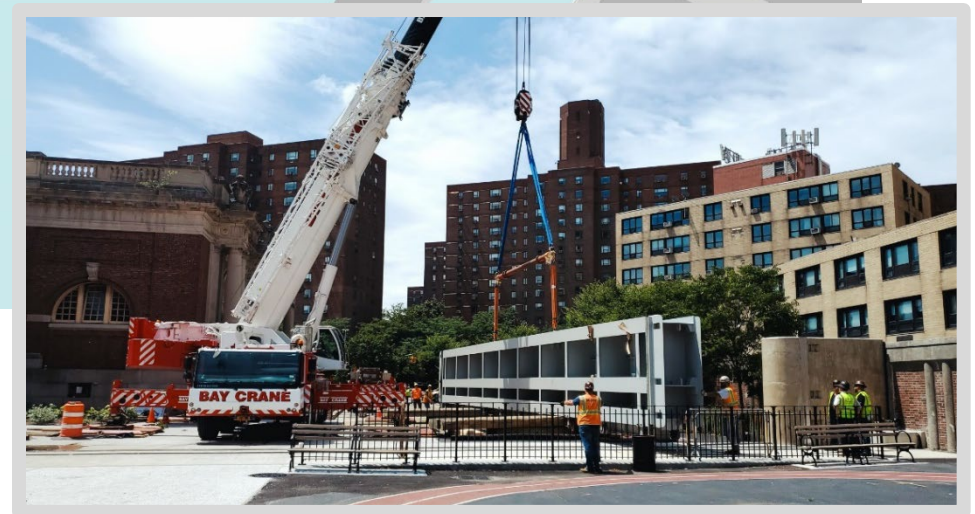
Floodgate 18 installed at Asser Levy Playground
