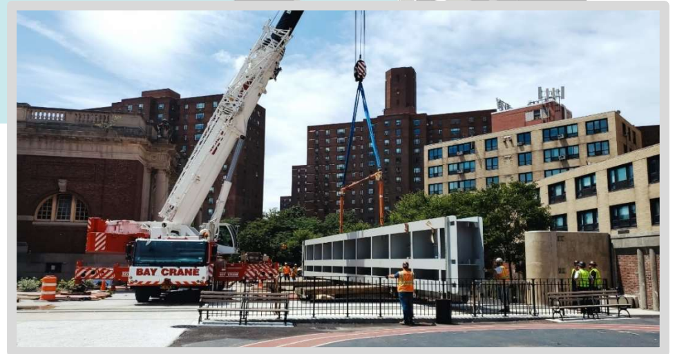
Floodgate 18 installed at Asser Levy Playground
