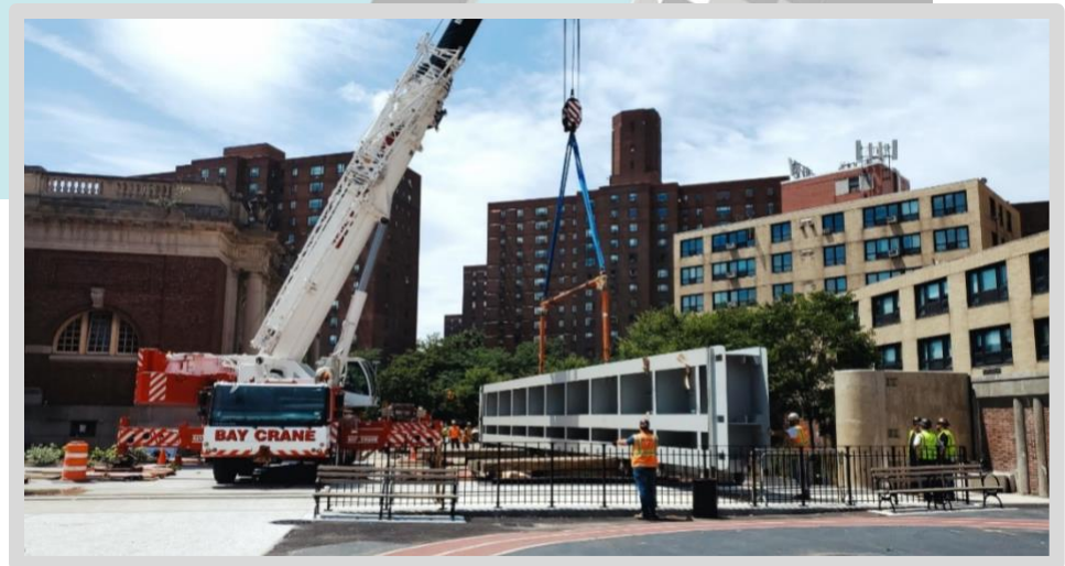
Floodgate 18 installed at Asser Levy Playground
