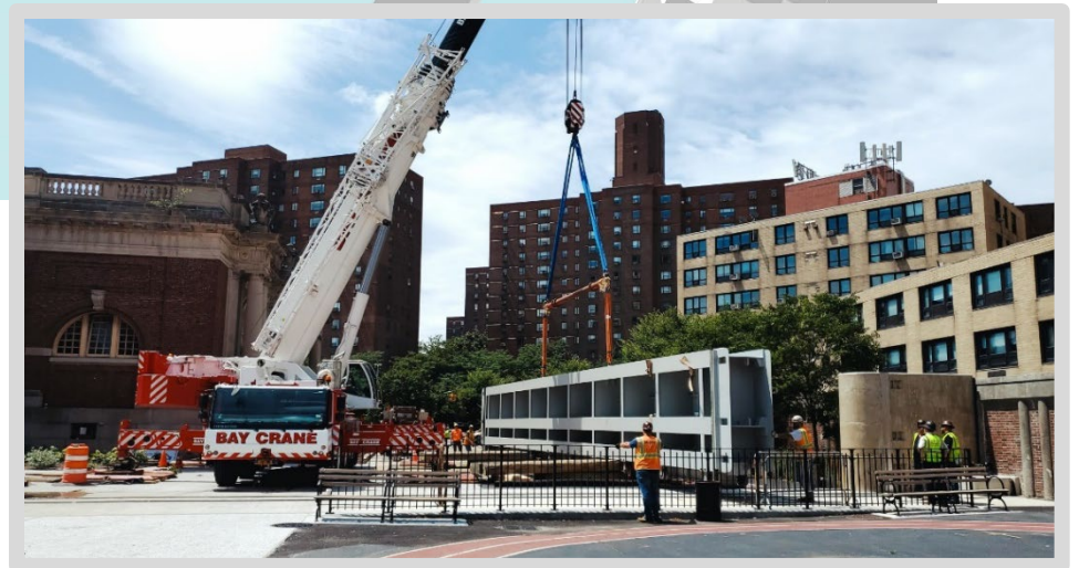
Floodgate 18 installed at Asser Levy Playground
