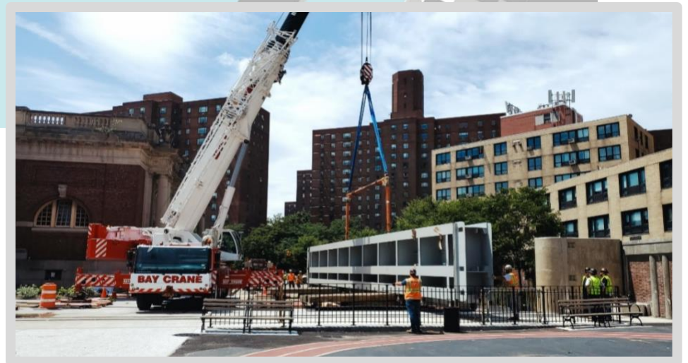
Floodgate 18 installed at Asser Levy Playground
