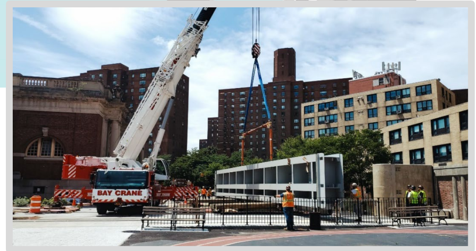
Floodgate 18 installed at Asser Levy Playground
