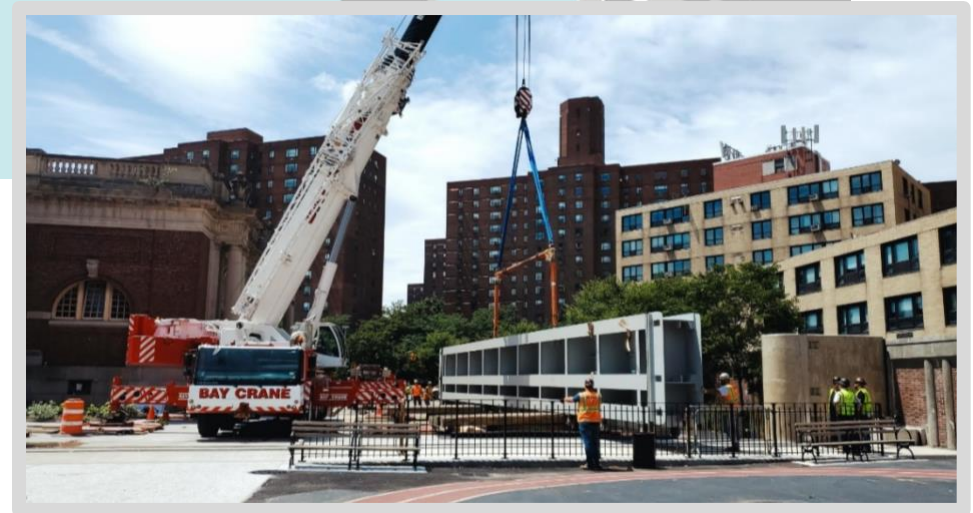
Floodgate 18 installed at Asser Levy Playground
